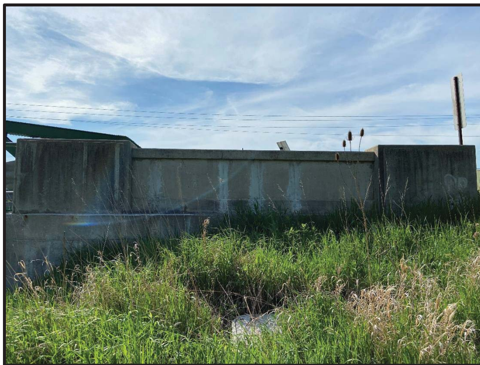
Image 23: Detail of Northwest Barrier Wall and North Wing Wall (May 27, 2020; View looking Southeast)
