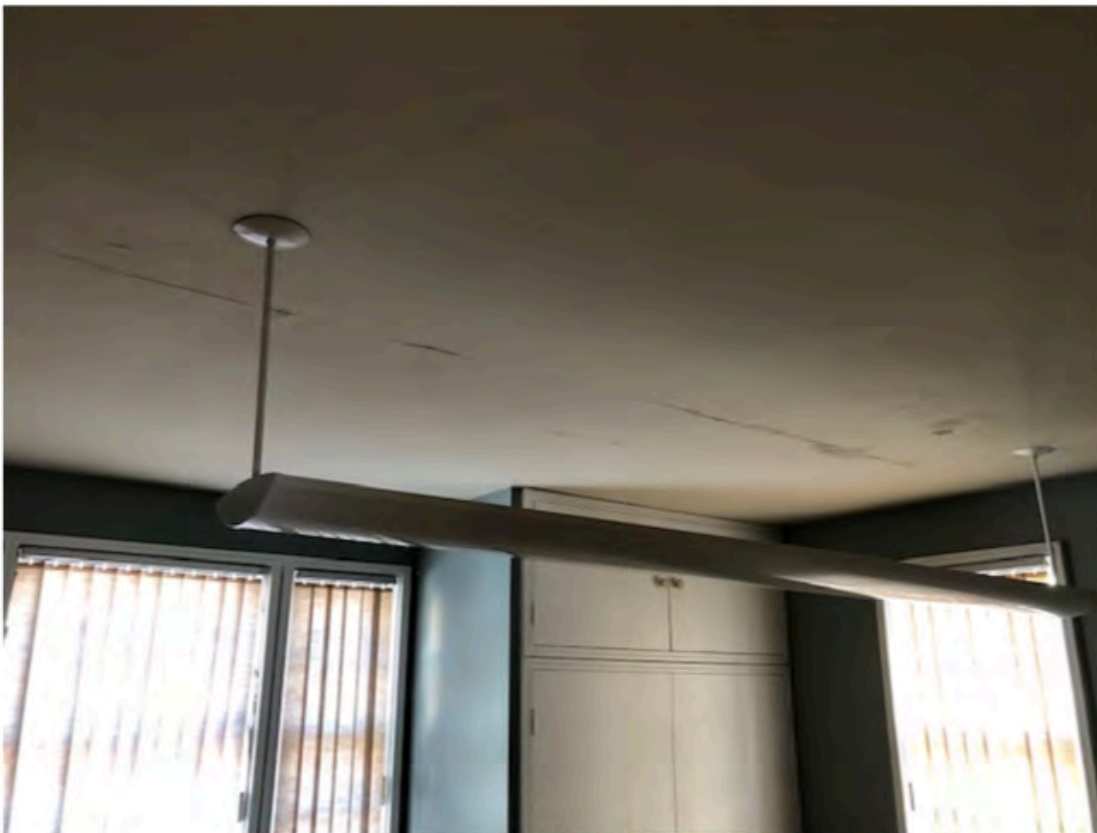
Ceiling damaged due to roof leaks - West wing office
