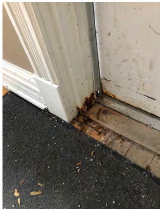
Deteriorated steel frame and door - West entrance
