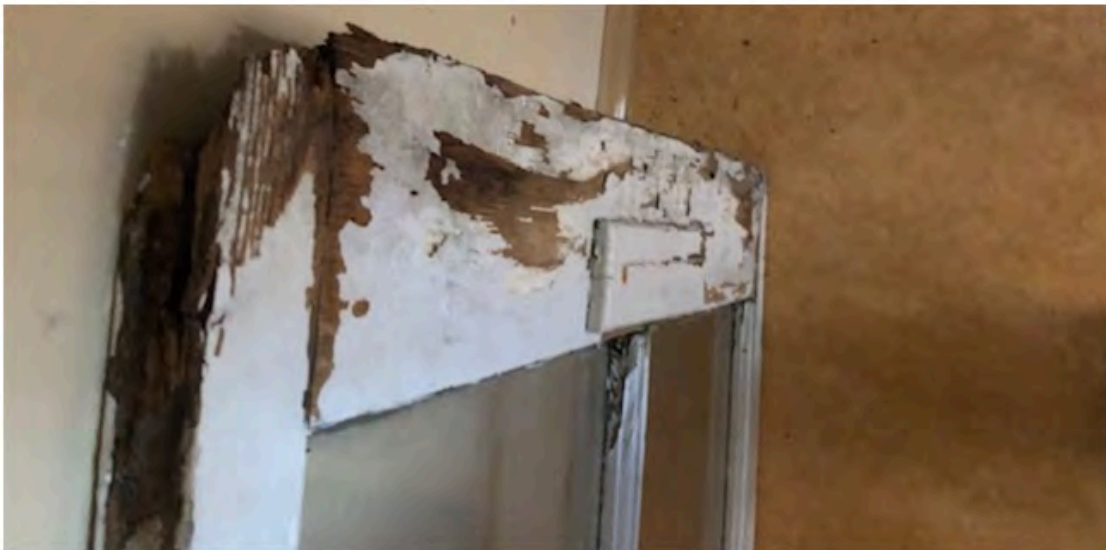
Storm window - Deteriorated bottom rail
