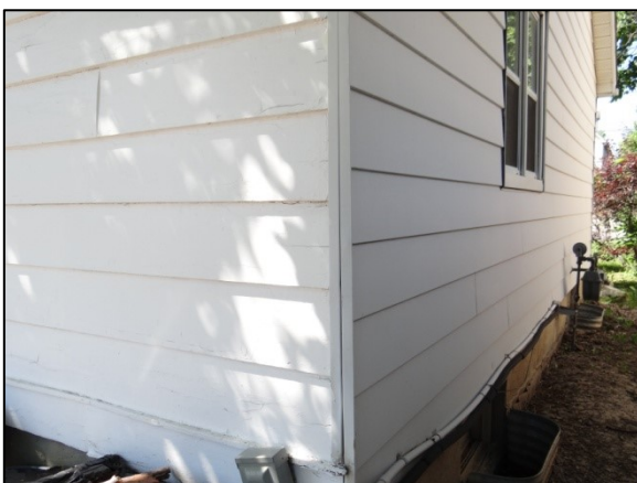
Figure 27: Clapboard on the northeast elevation and aluminum siding on the northwest elevation.
