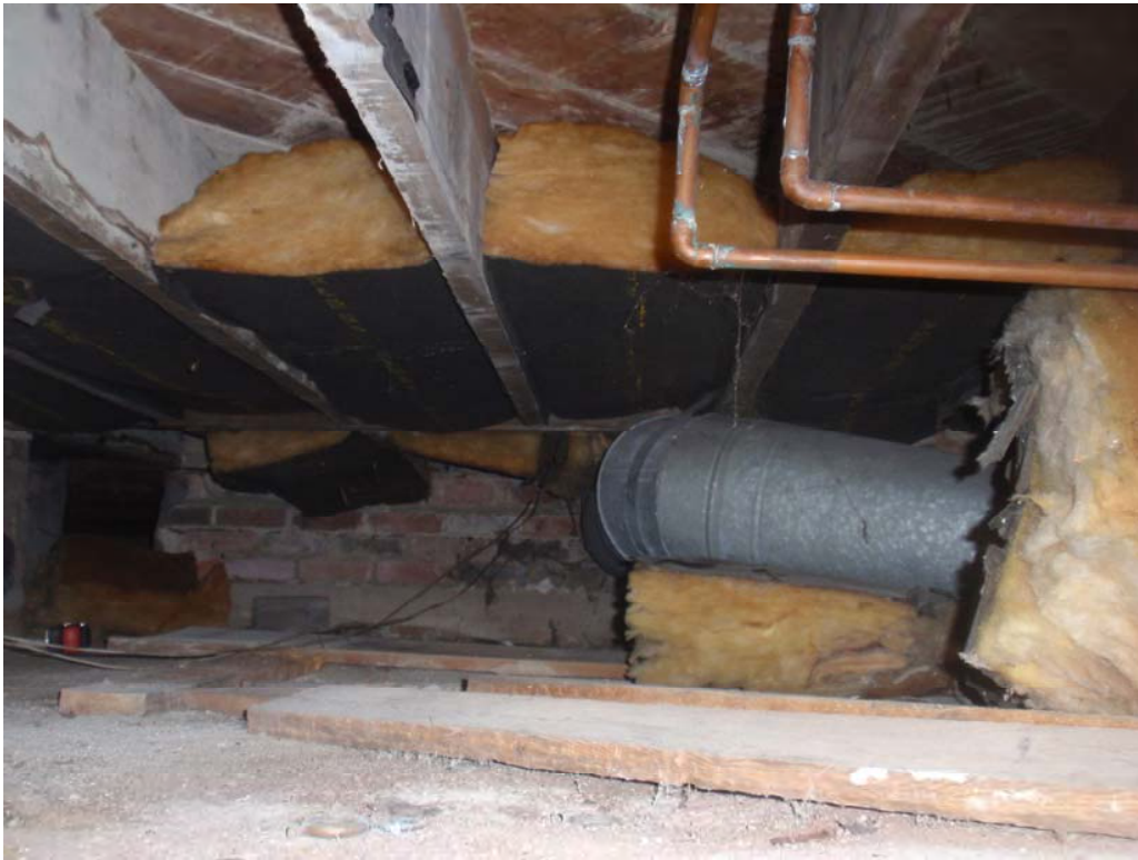
West Part of Basement (2-2x10 beam)
