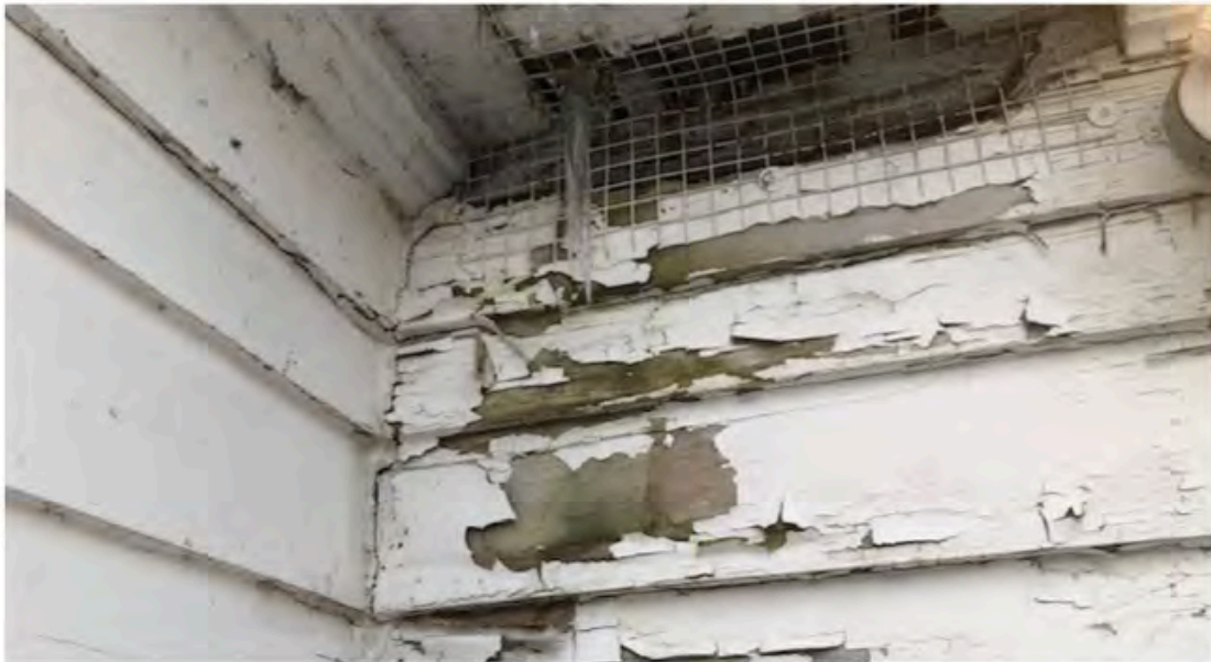
Deteriorated soffit, frieze and siding - West wing north elevation
