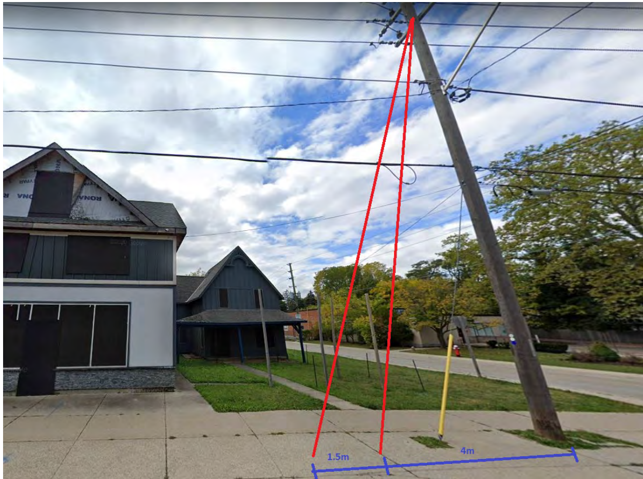
Figure 55: Sketch of the 2 new anchors to be installed on the existing pole in front of the property to provide structural stability, overlayed on the current conditions at 1140 Clarkson Rd N. (Source: CIMA+)
