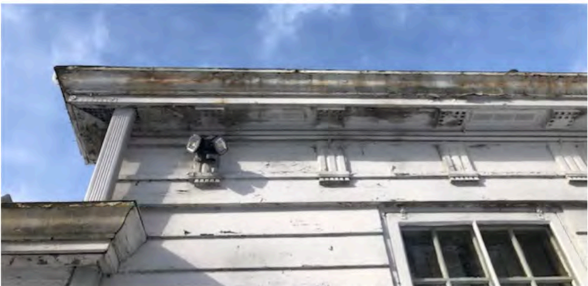
Frieze board with the Triglyph detail – Central part of the building south elevation
