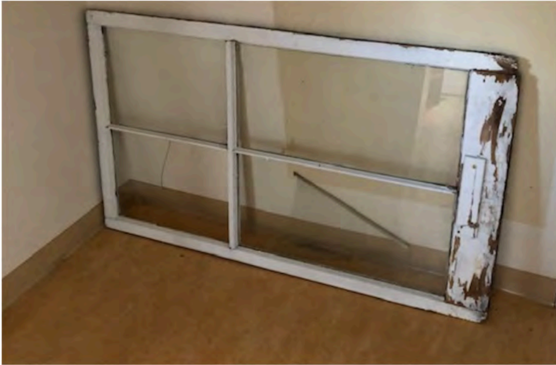
Storm window - Deteriorated bottom rail - south elevation
