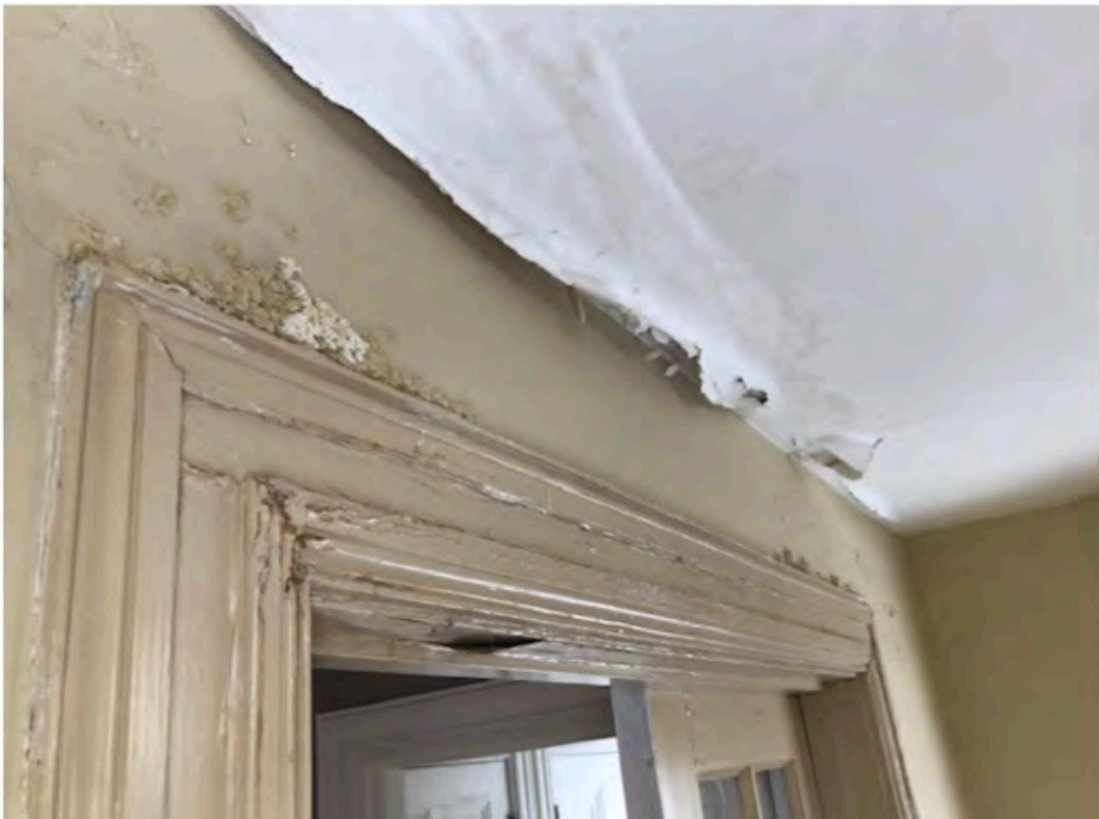
Ceiling damaged due to roof leaks - Main entrance vestibule
