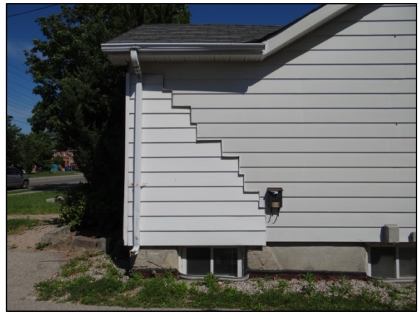
Figure 26: Repairs to the siding and the transition from lined to smooth parging on the foundation.
