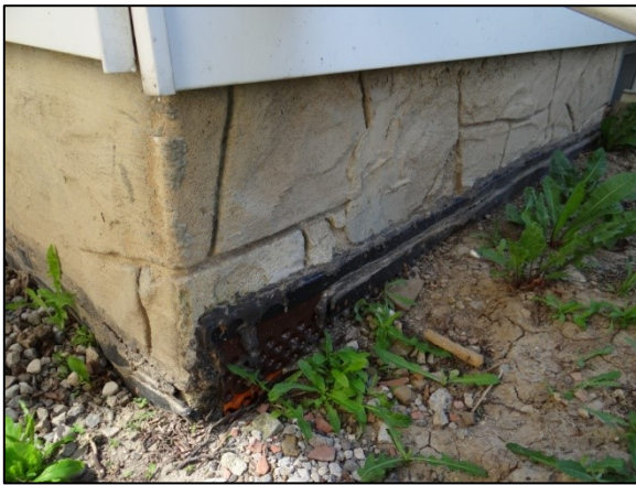
Figure 25: Lined parging along the foundation
