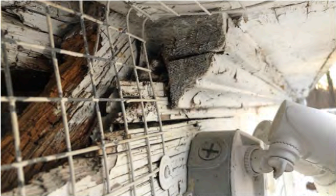
Deteriorated soffit, frieze and siding - West wing north elevation
