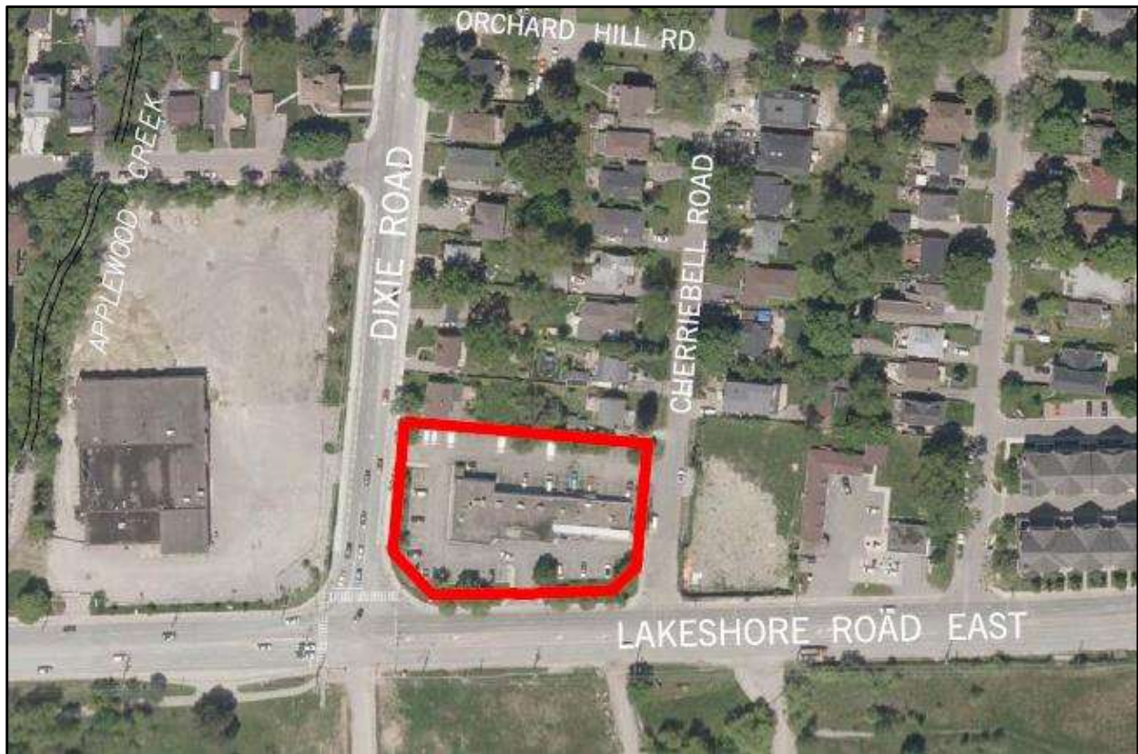
Aerial image of 1381 Lakeshore Road East
