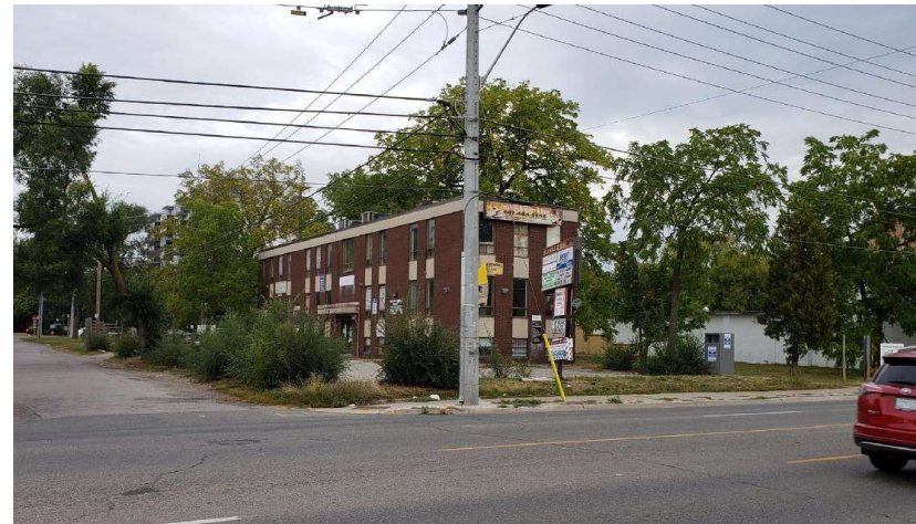
Subject Land – Looking northerly along Dundas Street West
