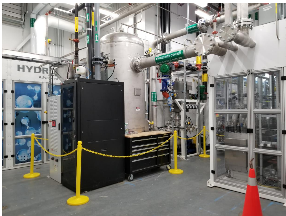
Figure 4: On-site Enbridge Hydrogen Production. Cabinet that houses the electrolyzer is shown on the right. Black box houses a fuel cell for low power lighting. Hydrogenics box contains dryer tank for final cleaning up of hydrogen.
