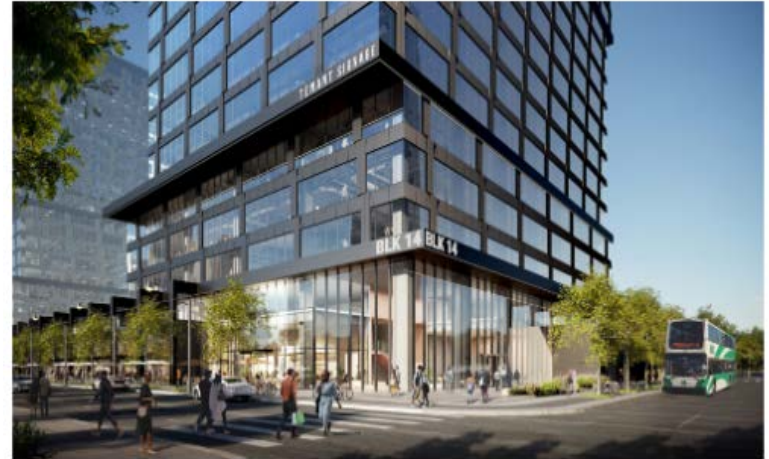
ARTIST RENDERING - MAIN ENTRANCE VIEW FROM INTERSECTION OF STATION GATE AND NEW STREET
