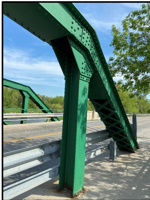
Image 8: End Post Detail, South Side of Old Derry Road Bridge (May 27, 2020; View looking North)
