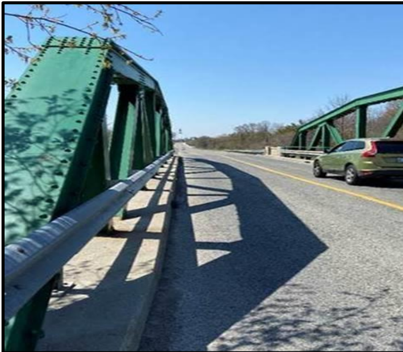
Figure 7: Existing Guiderail affixed to the Truss Members (McIntosh Perry 2021)
