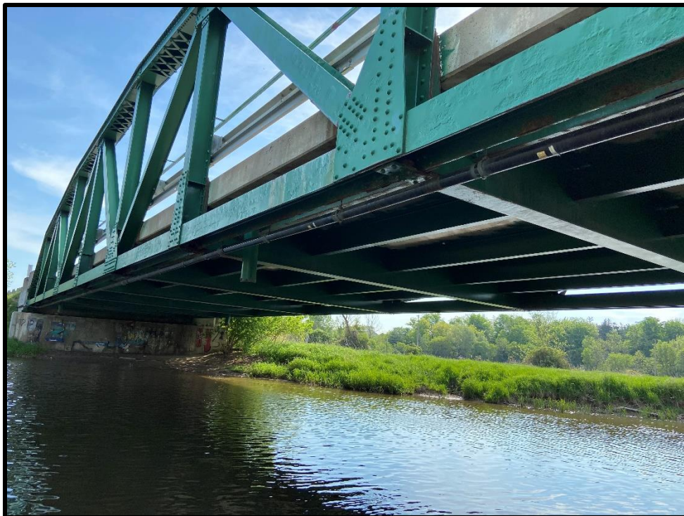
Image 28: Detail of Floor Beams and Stringers, Underside of Old Derry Road Bridge (May 27, 2020; View looking Northeast)
