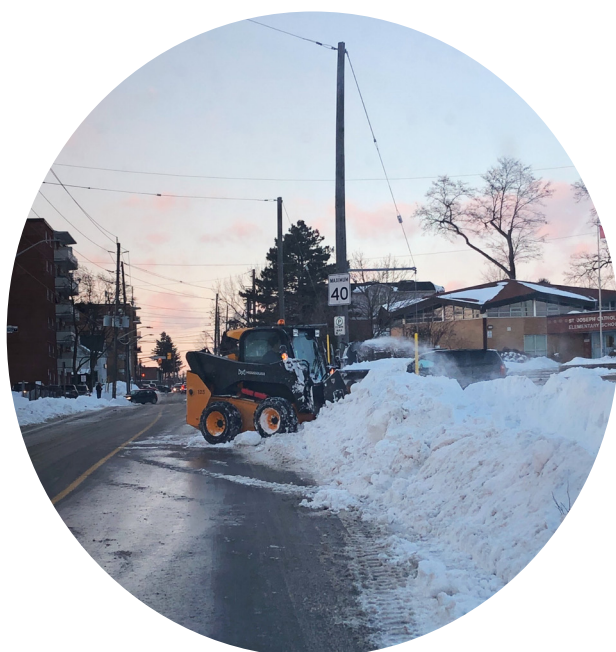
Crew clearing snow after a snow event – Action #60
