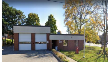
Fire Station Renovation Program
