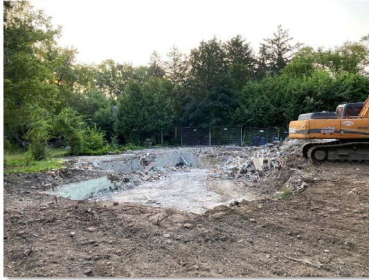
2515 Shepard Ave – Demolished
