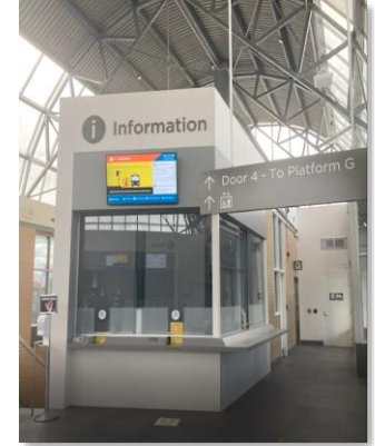
City Centre Transit Terminal Renovation
