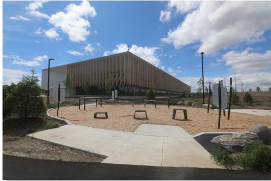
Rear Exterior View
