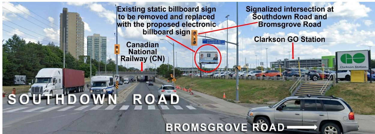
Image of the existing condition
