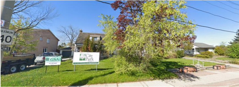
Images of existing conditions fronting Queen Street South (south half of the site)
