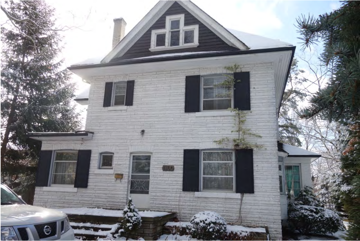
FRONT ELEVATION – re-clad with stone in the 1960s
