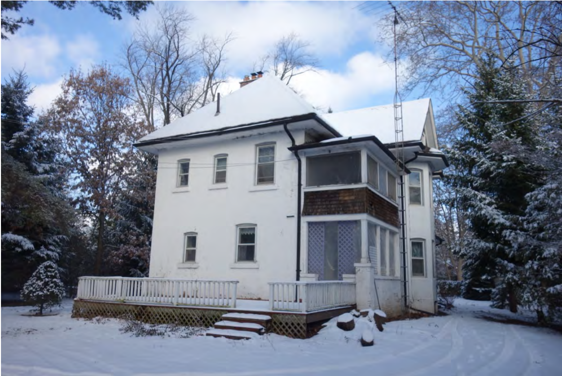
REAR & SIDE ELEVATION – the 2-storey screened sleeping porch – original wood shingles
