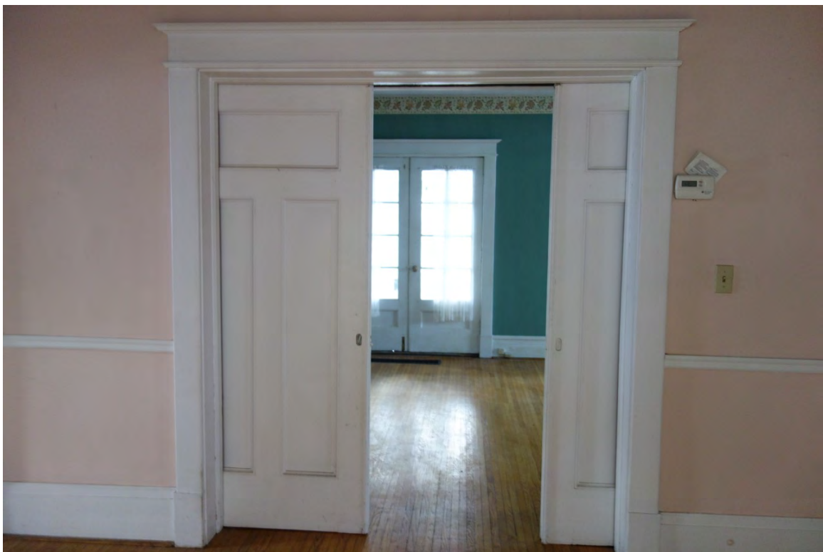
1 ST FLOOR – pocket doors between the living room and dining room
