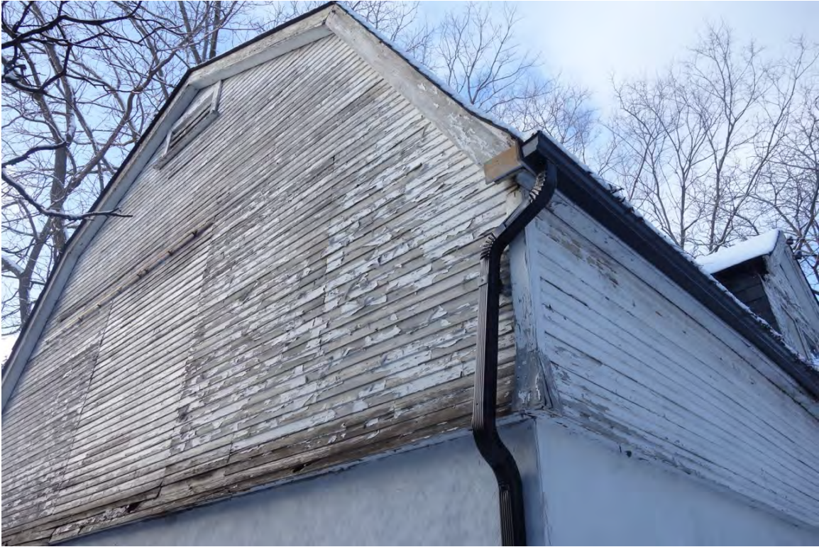
GARAGE – narrow wood siding with a subtle flare at the lower corner
