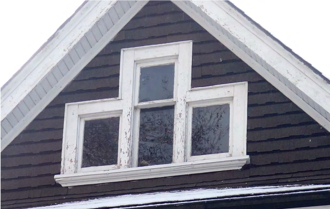
FRONT GABLE – wood shingle replaced (or covered?) with asphalt shingle
