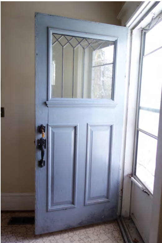
DOORS & WINDOWS – front door with leaded glass – segmentally arched masonry openings with concrete brick sills and lintels – wood sash window with modern aluminum storm
