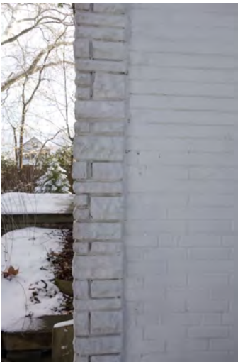
MASONRY DETAILS – the edge of the 1960s stone veneer at the corner of the façade (left) and the original 1913 cement brick (right)
