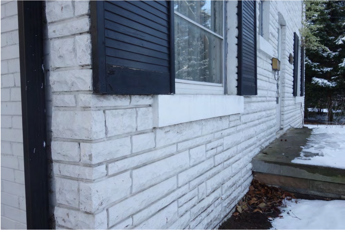
MASONRY DETAIL – front façade was re-clad with stone in the 1960s
