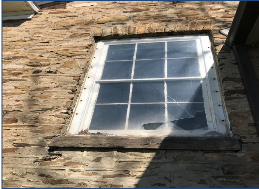
Damaged Plexi window pane recommended for replacement
