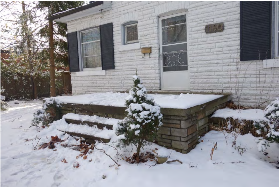
FRONT ENTRANCE – concrete stoop with stone veneer that replaced the original front porch
