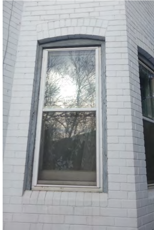
DOORS & WINDOWS – front door with leaded glass – segmentally arched masonry openings with concrete brick sills and lintels – wood sash window with modern aluminum storm
