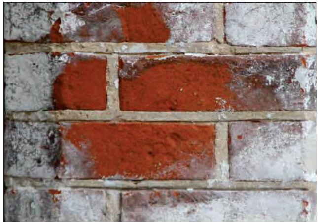
Figure 29 original red-orange brick under white paint
