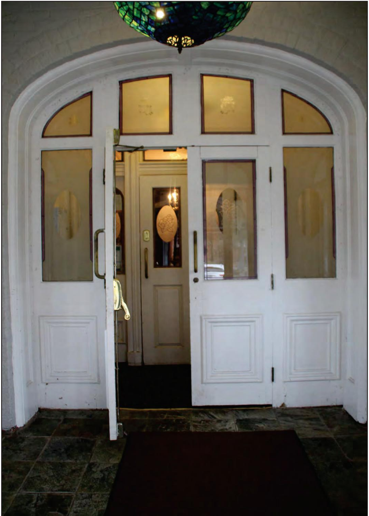
Figure 51 doors, top lights and sidelights (replacement glass & hardware) to umbrage from exterior
