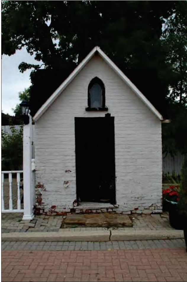
Figure 59 outbuilding - south facade
