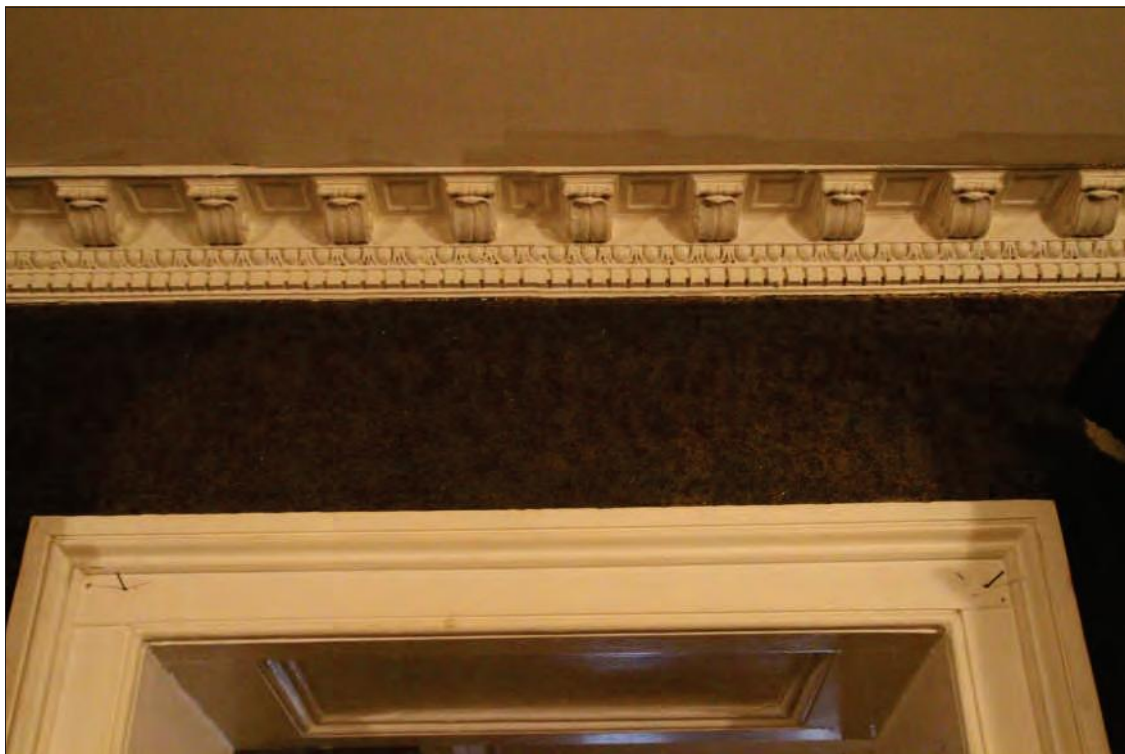
Figure 50 plaster ceiling moulding in current bar
