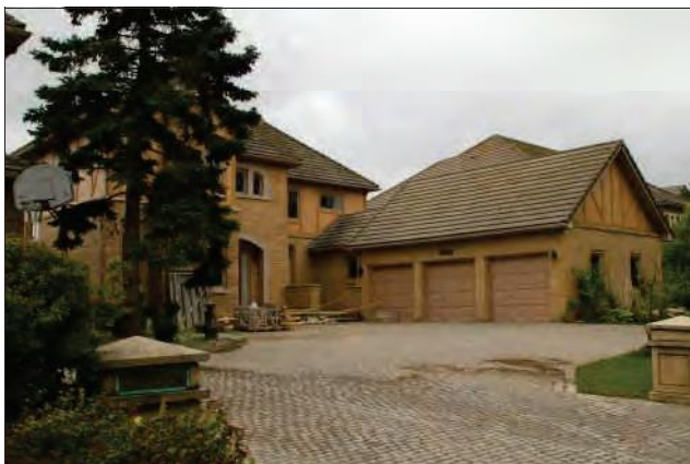
Figure 67 west side Mississauga Road
