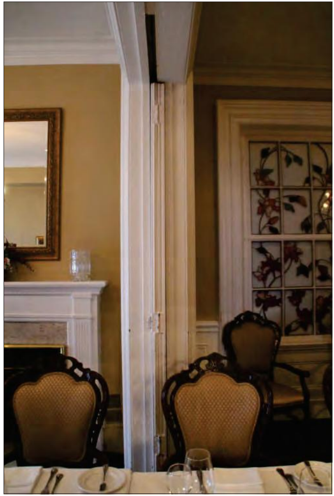
Figure 46 folding pocket doors between north parlours
