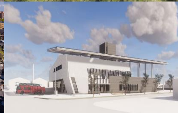
Vancouver Fire Hall No. 17
