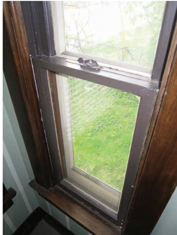
Detail of bay-window (ERA, 2022).
