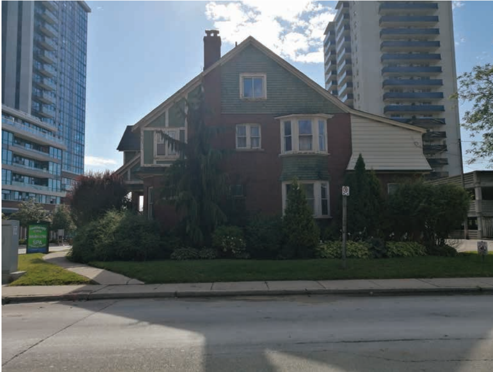
Looking southeast from the Site across High Street East (ERA, 2021).
