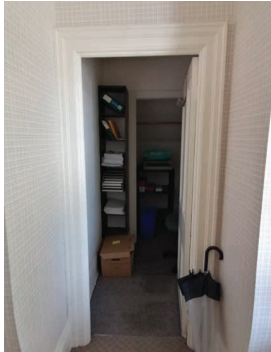
Second floor wood trim (ERA, 2021).
