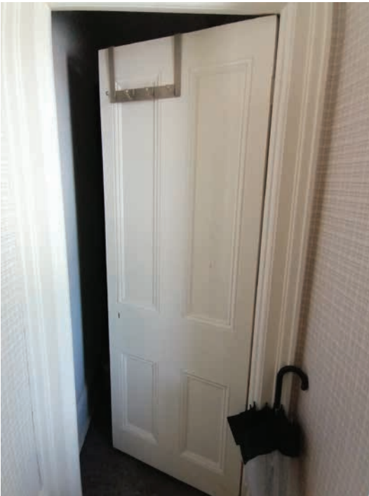
Second floor wooden four-panel door (ERA, 2021)
