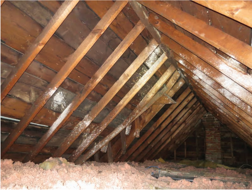
Attic looking east (ERA, 2022).
