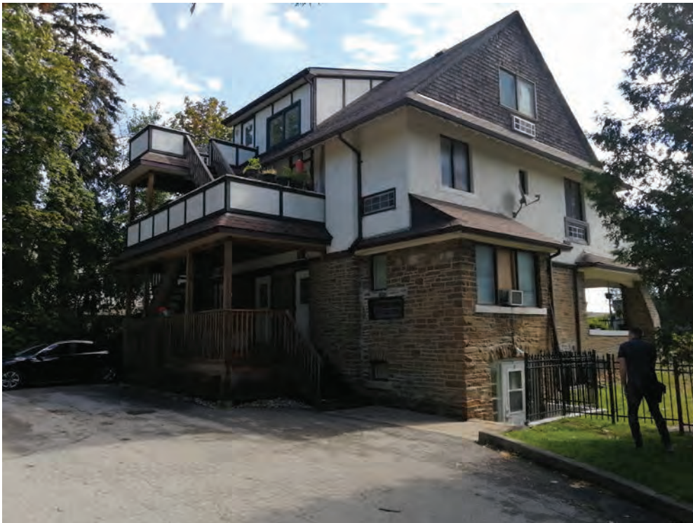
North and west elevations of 84 High Street East (ERA, 2021).
