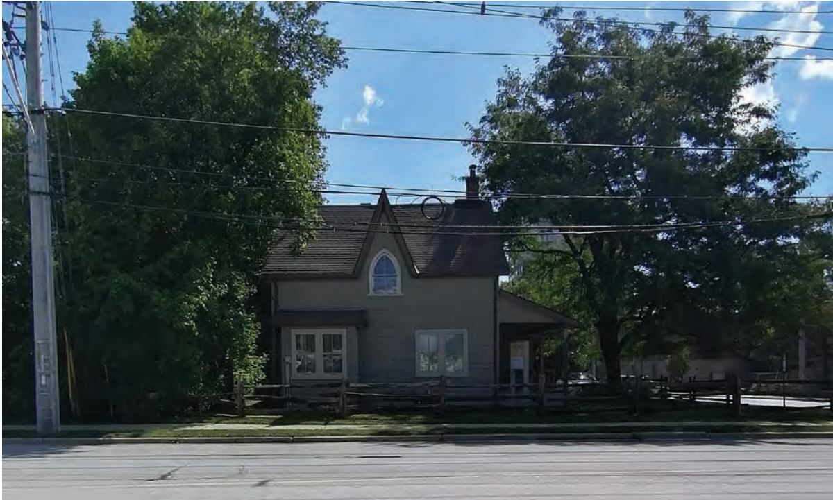
North elevation of 19 Ann Street (ERA, 2021).
