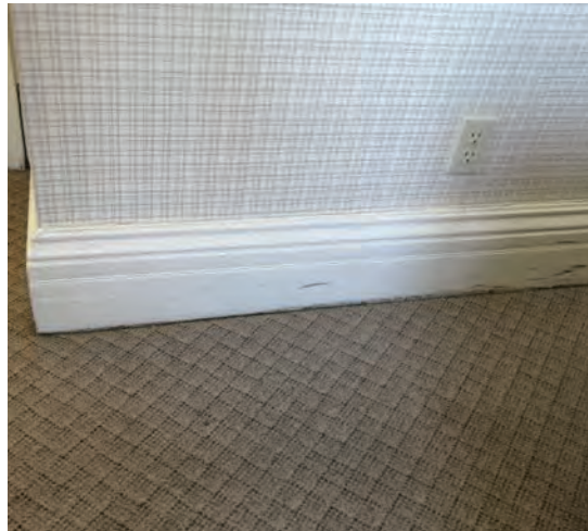
Second floor baseboard (ERA, 2021).
