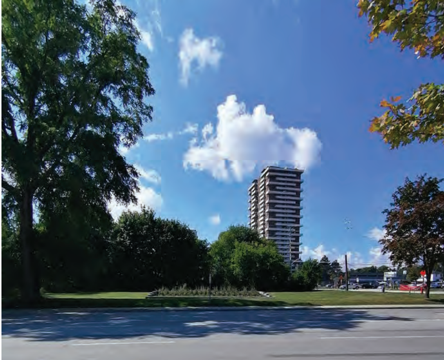
91 Park Street East from Hurontario Street (ERA, 2021).
