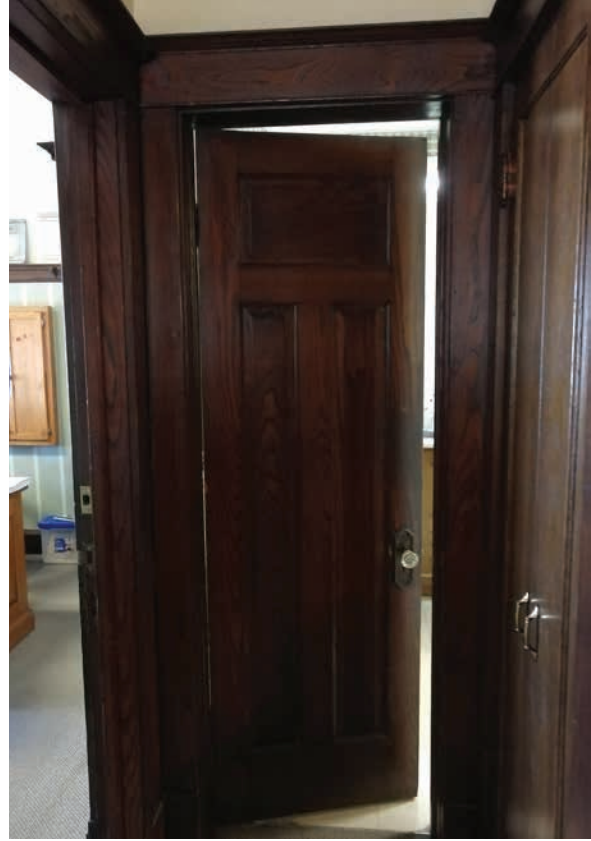
First floor hallway wood-panelled door and trim (ERA, 2021).
