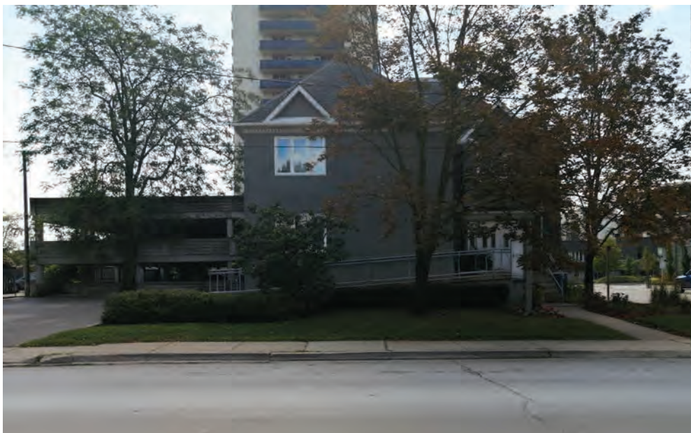
Looking southeast from the Site across High Street East (ERA, 2021).
