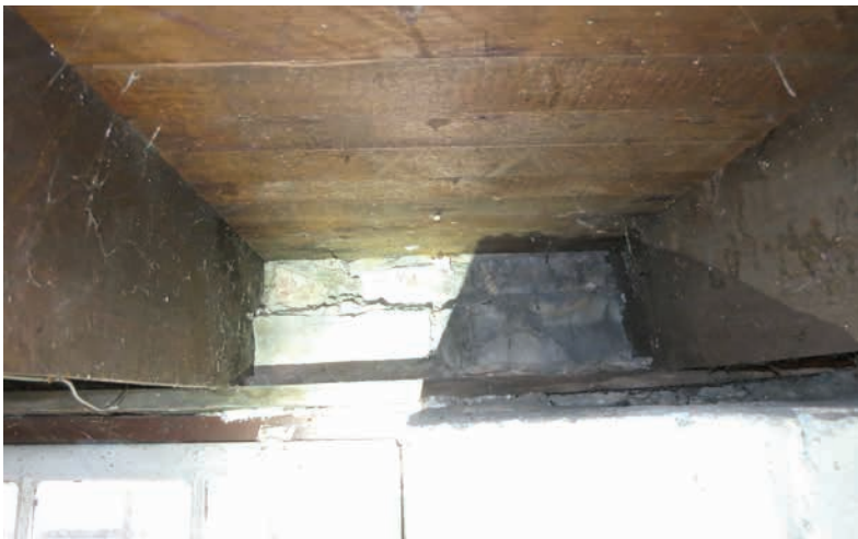
Top of foundation wall (ERA, 2022).
