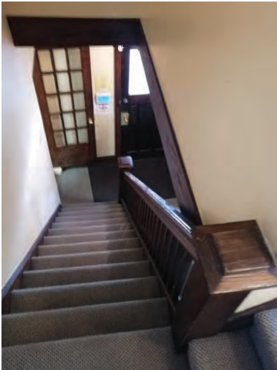
Staircase from second floor (ERA, 2021).
