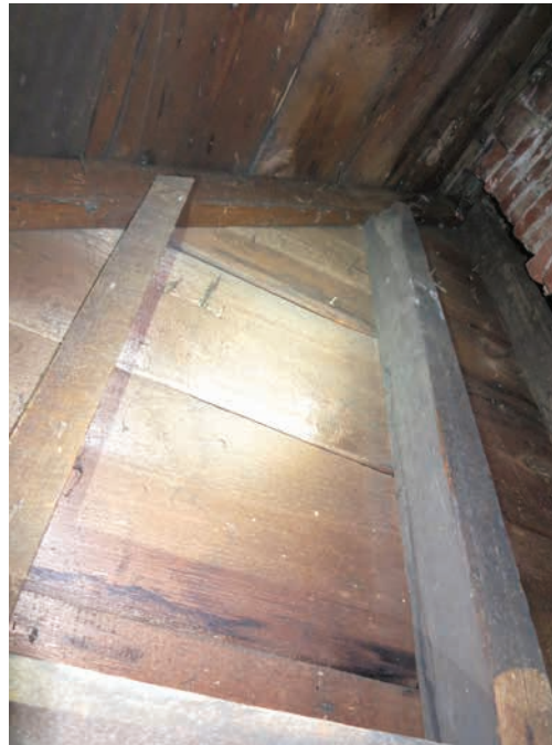
Attic detail of wooden cladding (ERA, 2022).
