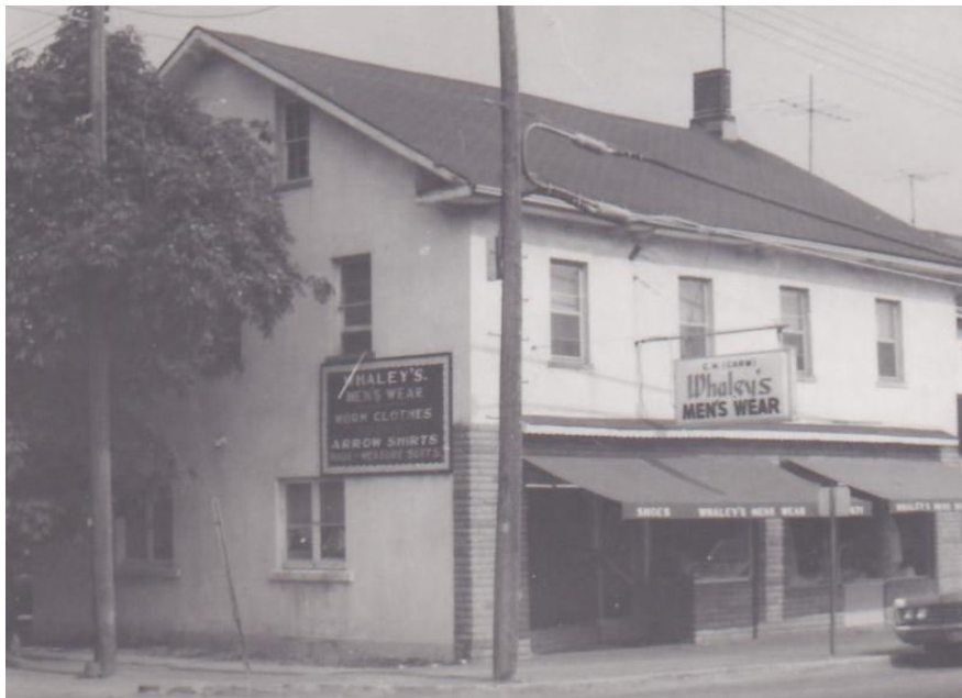
Historical image of 213 Queen Street South (photo credit: Streetsville Historical Society).
