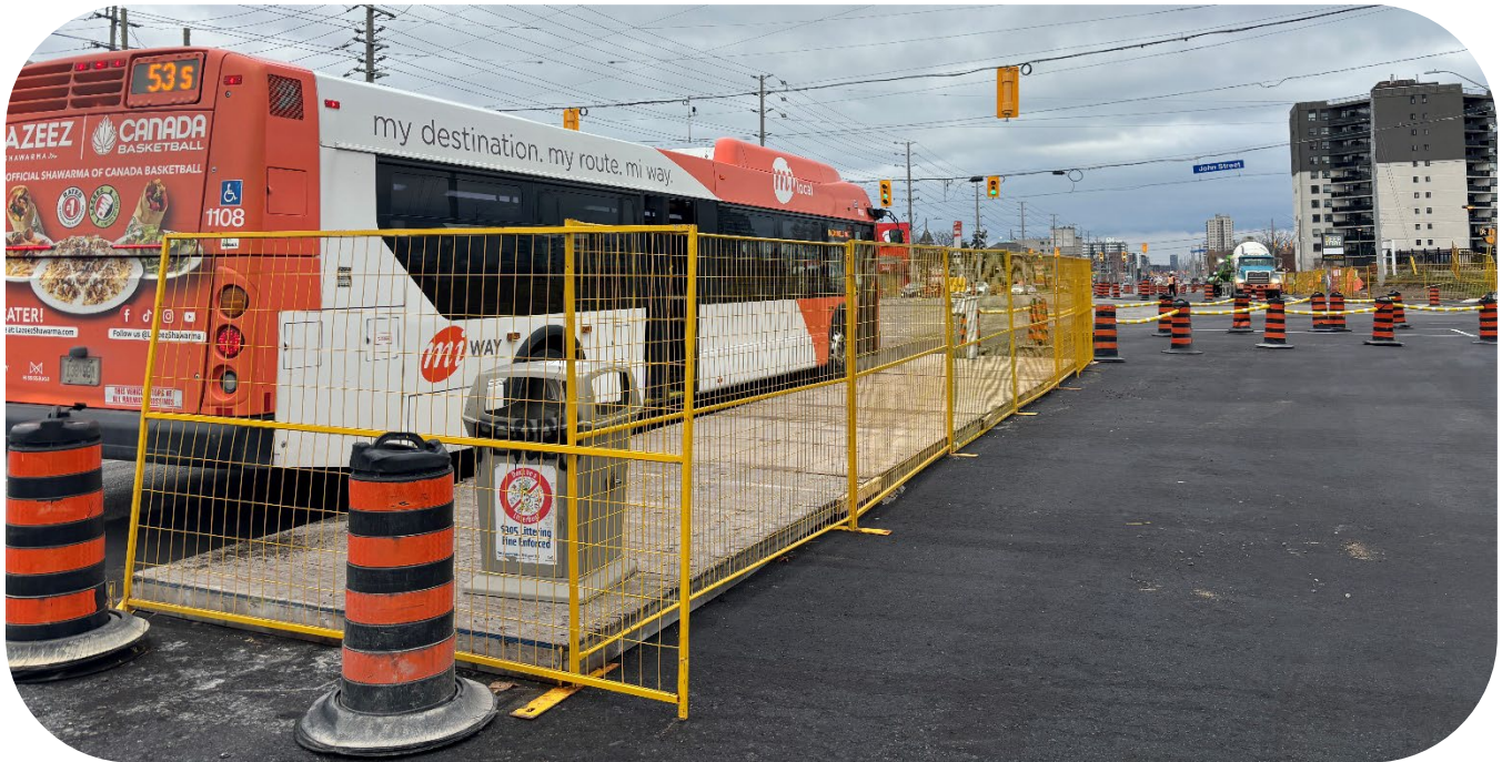
Figure 6: Temporary pedestrian landing pad platform.
