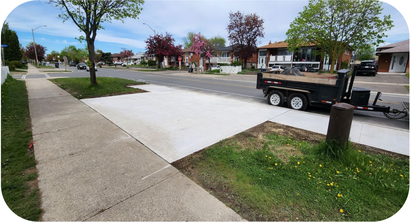
Figure 1: New customer landing pad and transit shelter pad at bus stop#2362 Morning Star Dr. at Netherwood Rd.
