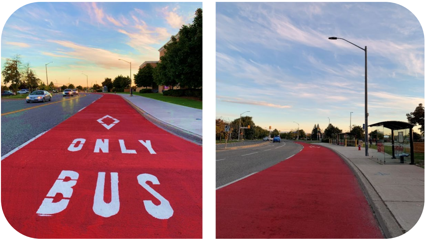
Figure 5: Laird and Vega Transit Terminal with the red surface treatment application.
