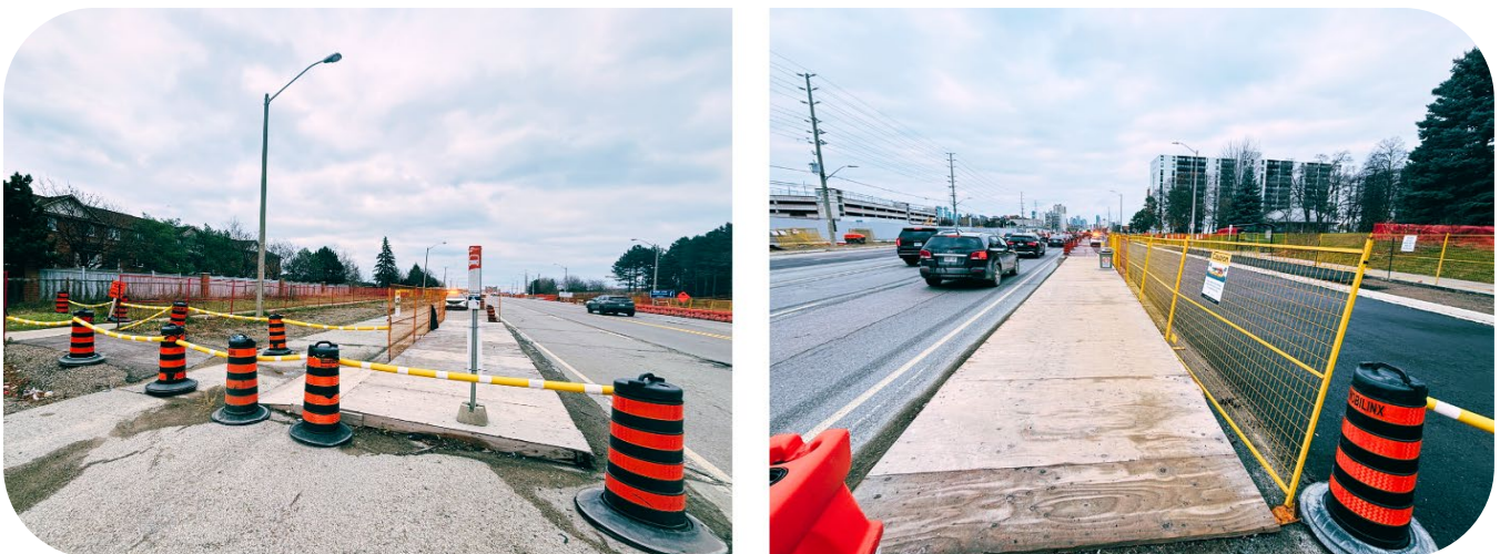
Figure 7: Temporary pedestrian walkways and ramps.
