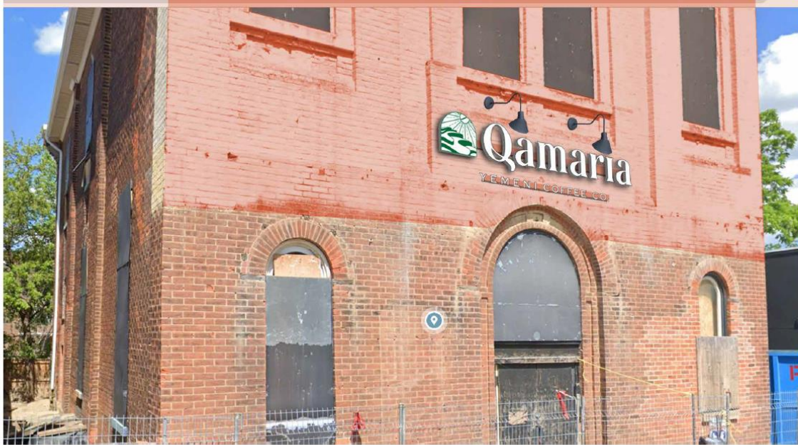
North Side Front Entrance
