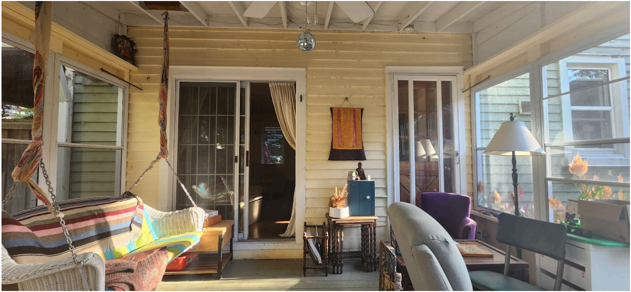
Figure 6: Interior view of rear sunroom, showing the existing rear wall of the house with existing swing and sliding doors. (Photo by owner, October 2024)
