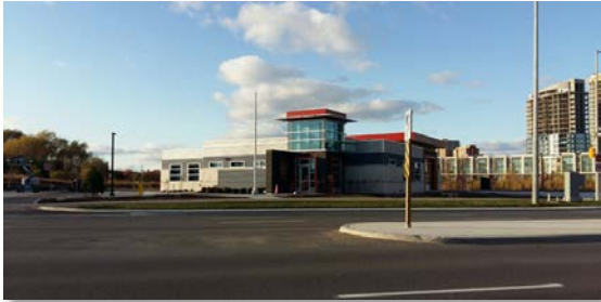
New Fire Station 120 opened at Hurontario and Eglinton
