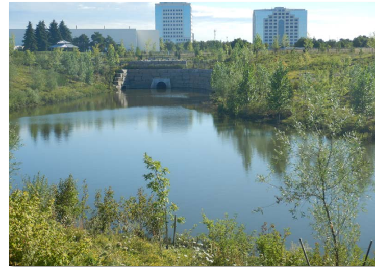
Storm sewer outfall into new Saigon Park stormwater management pond
