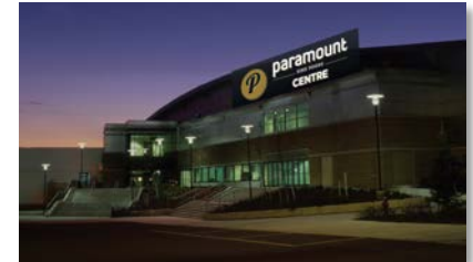
PARAMOUNT FINE FOODS CENTRE ARENA RENEWAL
