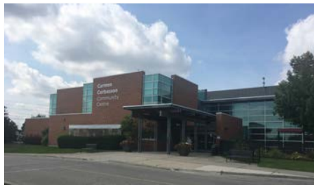
CARMEN CORBASSON COMMUNITY CENTRE REDEVELOPMENT
