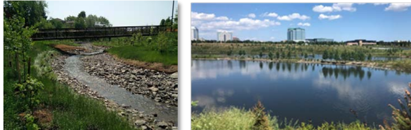
Flood and erosion control on Cooksville Creek
