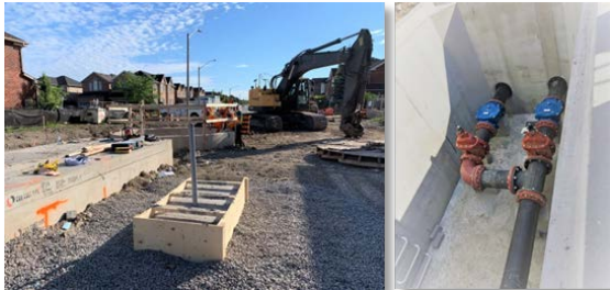
Lisgar pumping station construction
