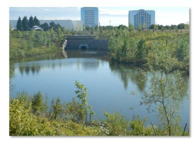
Storm sewer outfall into new Saigon Park stormwater management pond
