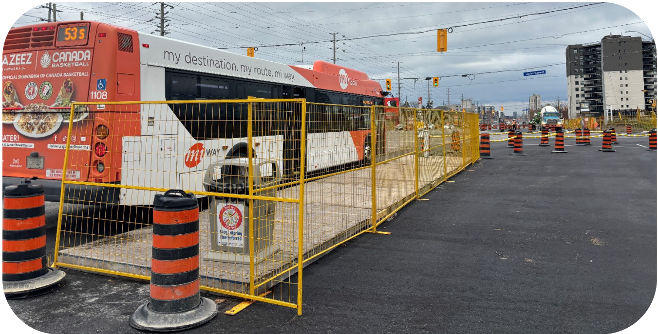
Figure 6: Temporary pedestrian landing pad platform.
