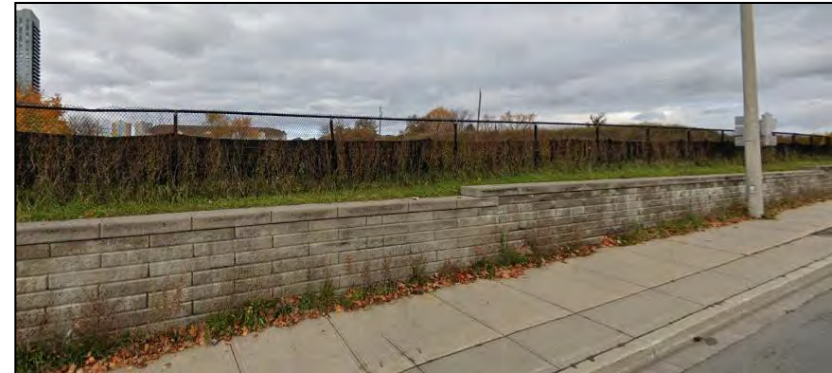
Example Major Retaining Wall
