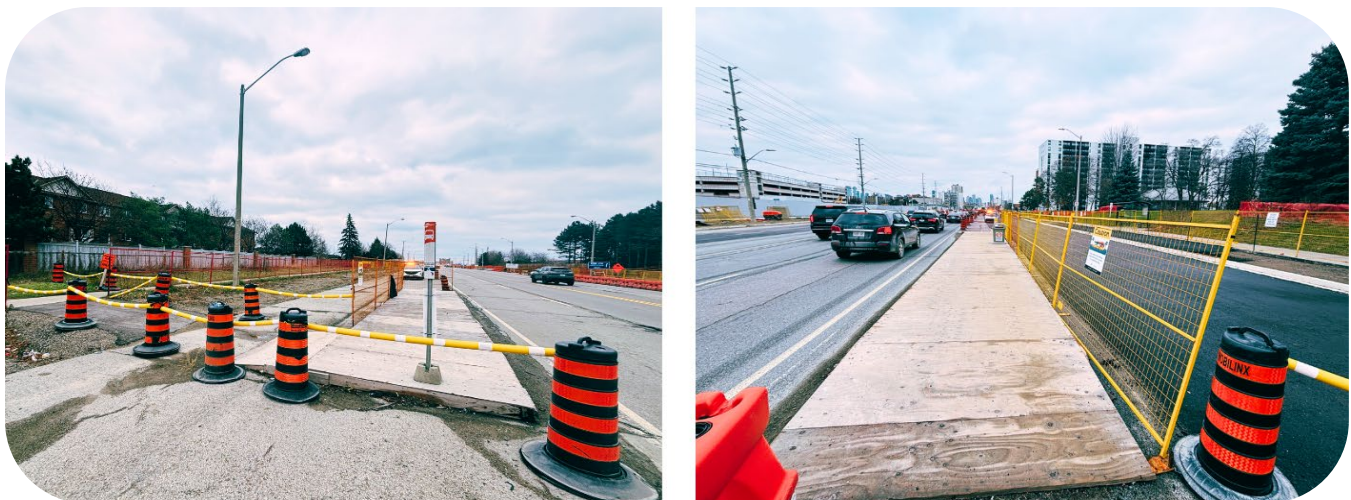
Figure 7: Temporary pedestrian walkways and ramps.
