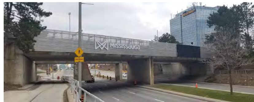
Example Rail Bridge
