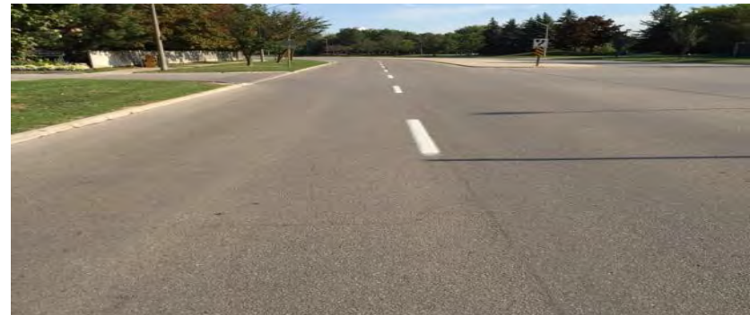
Road Pavement in Very Good Condition
