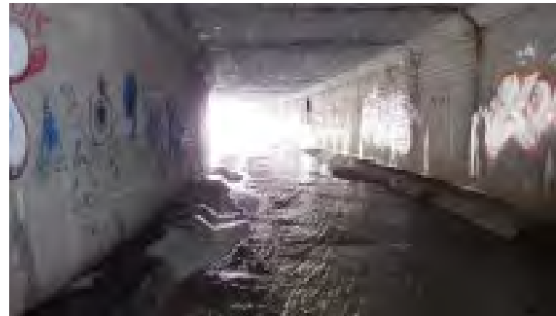
Trunk Storm Sewer under Dundas St. W
