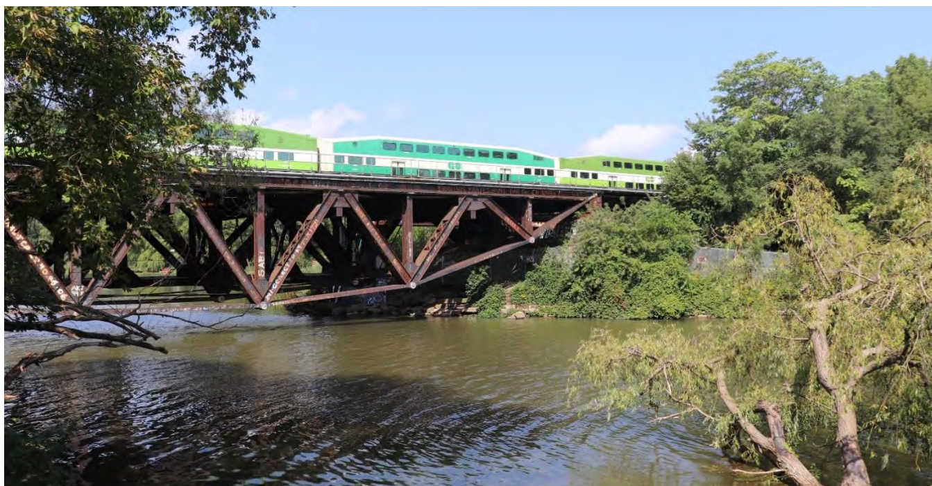
Photograph 3: View of the Credit River Bridge (Lakeshore West Rail Corridor), illustrating the Warren Truss configuration and the inverted bowstring arch, looking northeast (AECOM, 2023)
