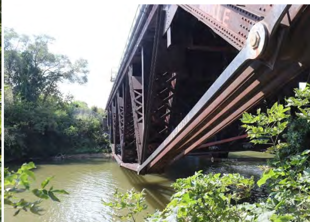
Photograph 3: View of the Credit River Bridge (Lakeshore West Rail Corridor), illustrating the Warren Truss configuration and the inverted bowstring arch, looking northeast (AECOM, 2023)
