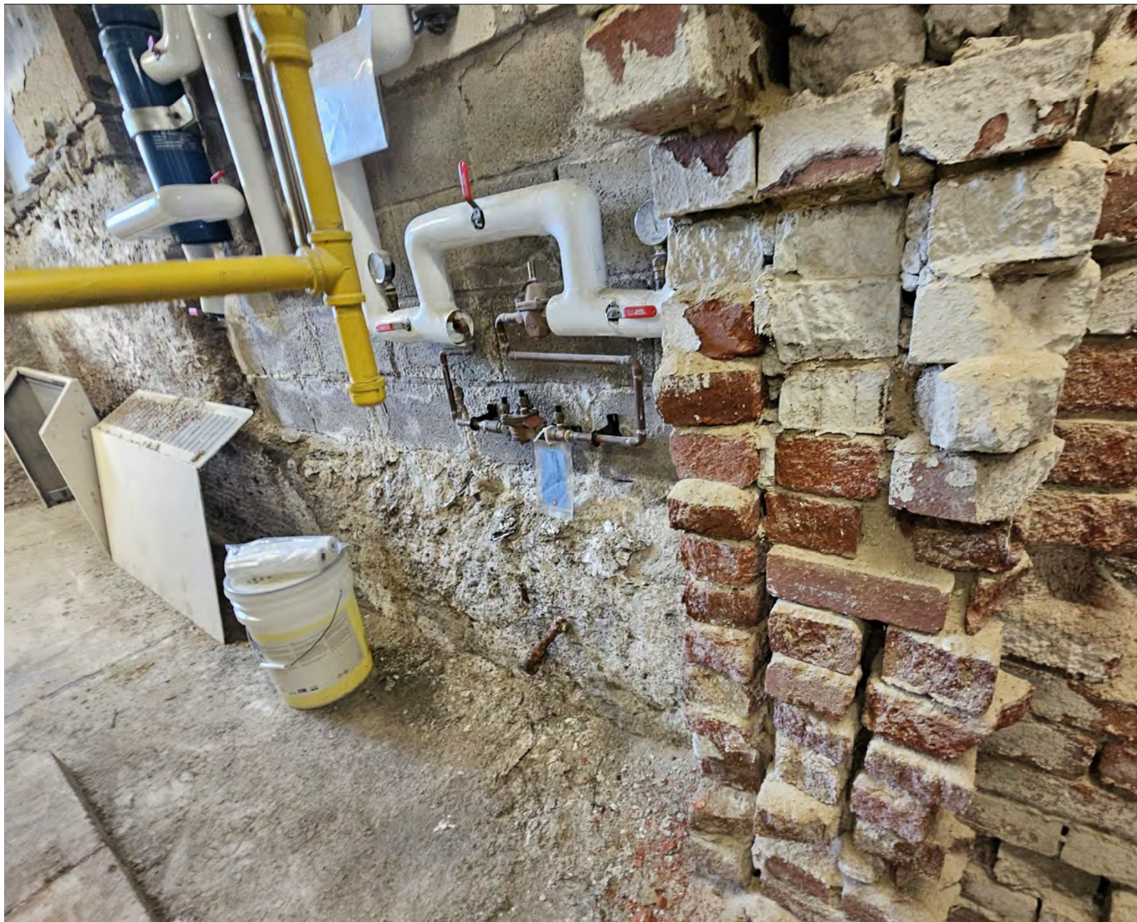
10 UTILITY ROOM - EAST WALL CONCRETE INFILL A2.1a NTS
