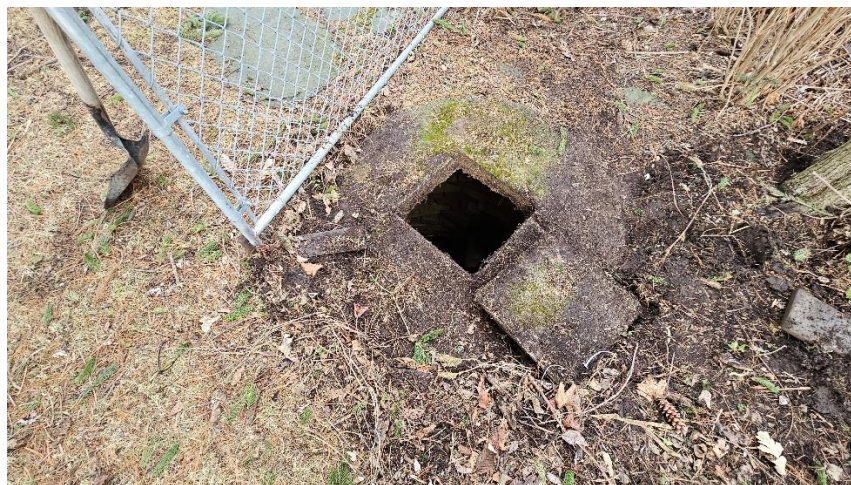
Photograph 6: Cistern Exterior Surface
