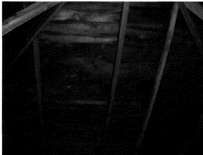
Inadequate and randomly spaced rafters
