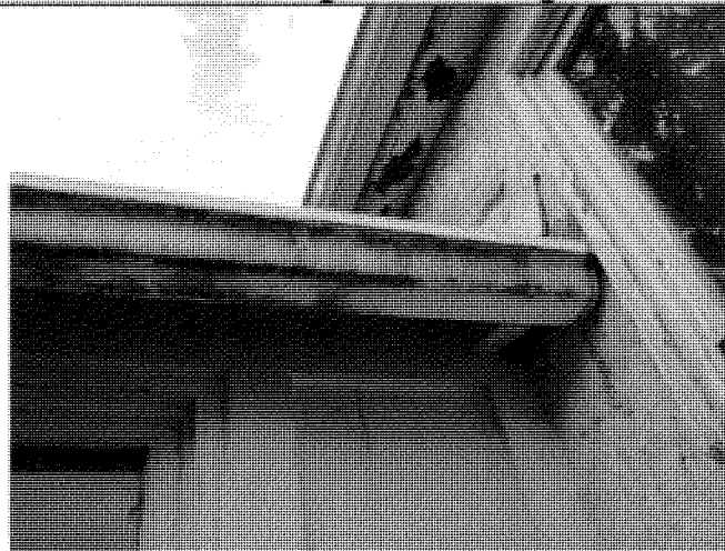
Photo 10: Poor drainage at Eavestrough
