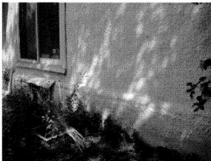
Misaligned foundation at rear wall
