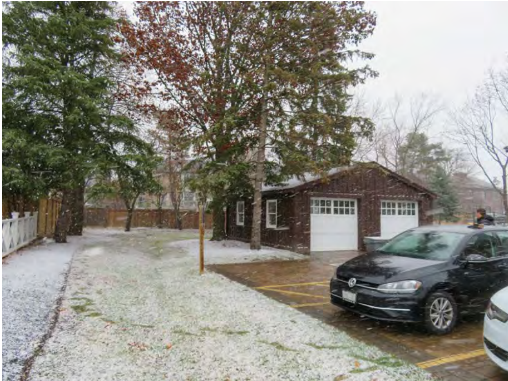
REAR YARD – non-historic outbuilding to be demolished
