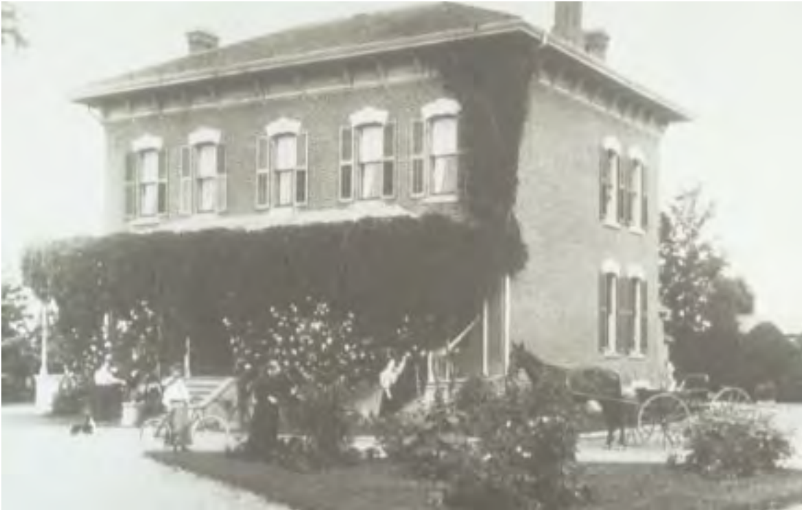
Gooderham Mansion, 929 Old Derry Road - built c.1870 for C.H. Gooderham (1844-1904)
