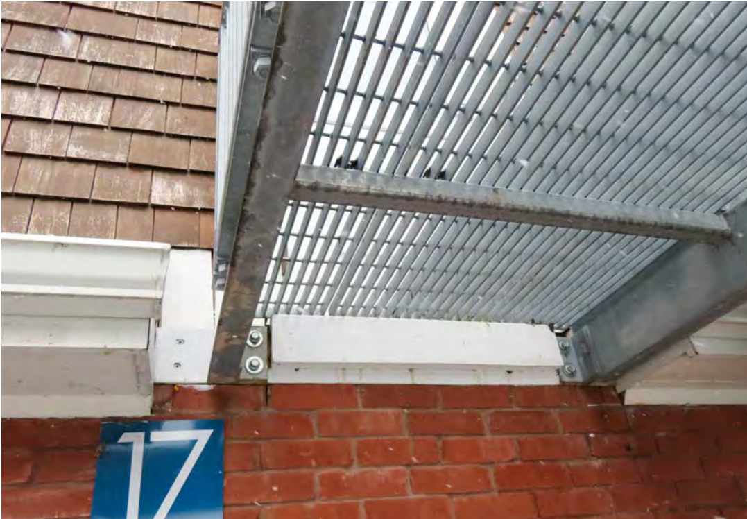
REAR ELEVATION – external fire exit stair from the 3 rd floor is to be removed – it is bolted into the masonry
