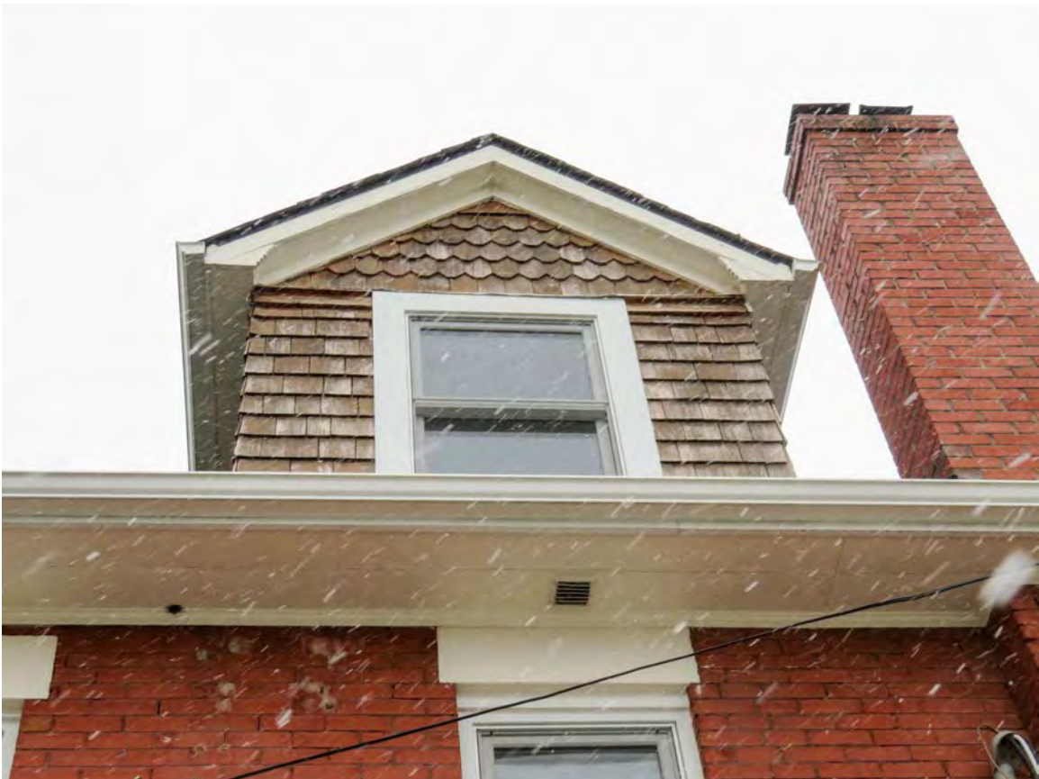
ROOF DORMER & BRICK CHIMNEY – the roof has a wide overhang – the wood shingles on the dormer are not original
