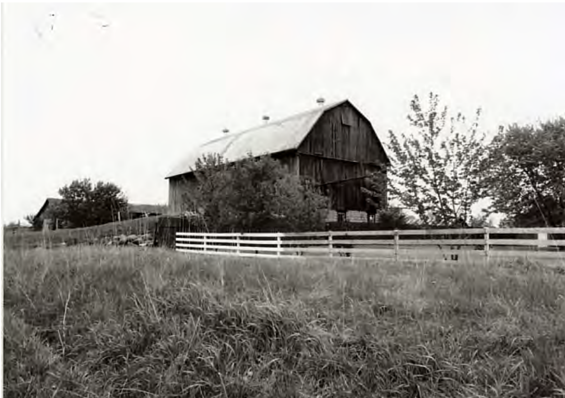
Gooderham barn, probably built c.1880 – one of several outbuildings on the estate
