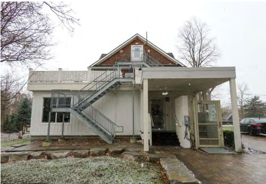
REAR ELEVATION – REAR ADDITION WITH METAL FIRE EXIT AND WHEELCHAIR LIFT TO BE DEMOLISHED
