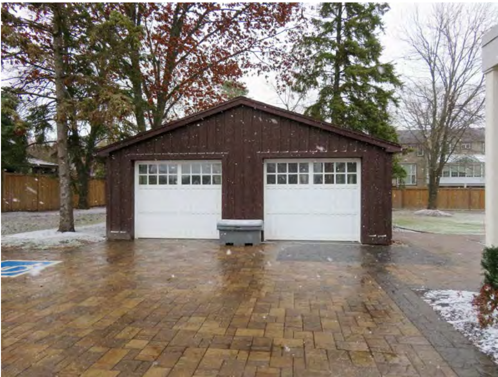
GARAGE – TO BE DEMOLISHED – a modern structure that has no cultural heritage value - concrete pad foundation – board & batten siding, aluminum doors - date of construction estimated to be c.1970s or 1980s
