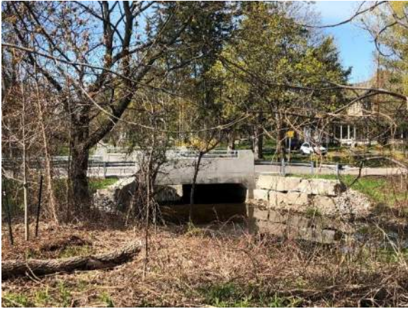
Image 21: View of the armor stone retaining walls on the east side of the culvert
