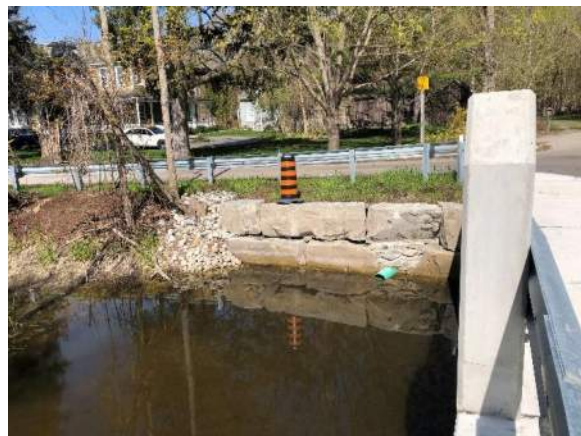
Image 20: View of armor stone retaining wall at the northwest corner of the culvert
