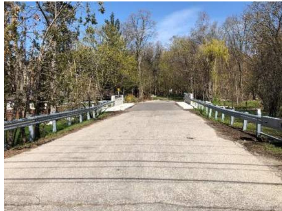
Image 18: View of new barrier systems along the south approach to the culvert
