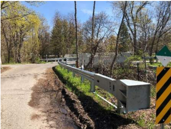
Image 17: View of new barrier systems along the north approach to the culvert
