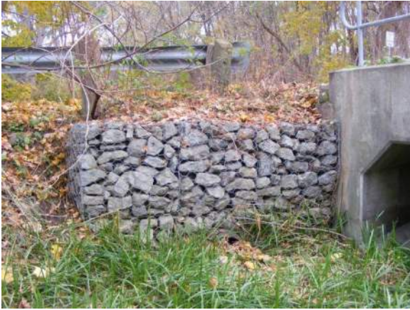
Image 8: View of gabion to the northwest corner of the culvert (City of Mississauga, 2007)
