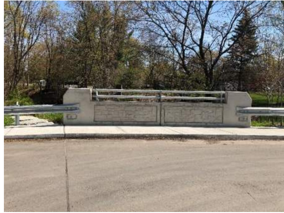
Image 16: View of the replaced pedestrian railing on the east side of the culvert
