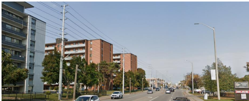
Looking east along Lakeshore Road East (mid-rise apartment on north side and strip commercial uses on south side)
