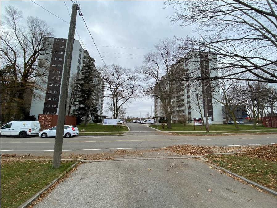
Image of existing conditions facing west
