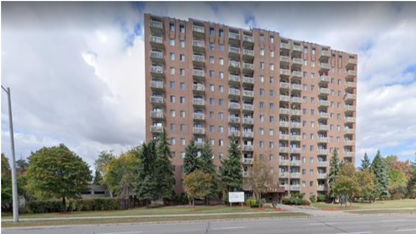
Photo from Aquitaine Avenue facing north
