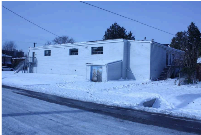
Figure 15 795 First Street, Mississauga, looking northwest, 2019. (Photo by author.)
