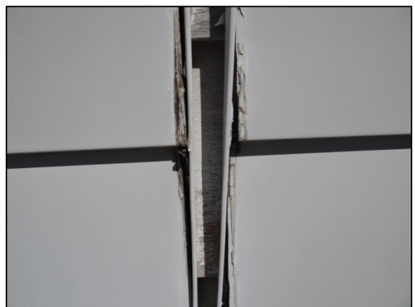
Figure 28: The original clapboard siding beneath aluminum siding.
