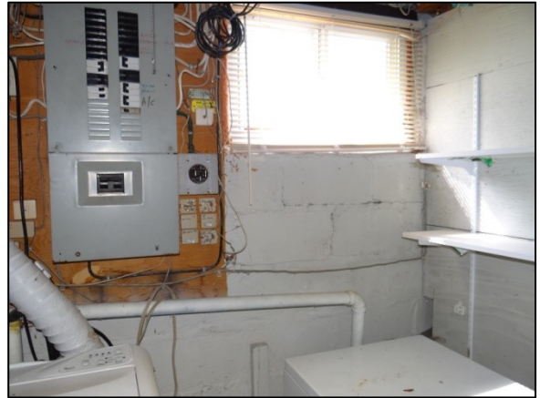
Figure 46: Concrete block foundation
