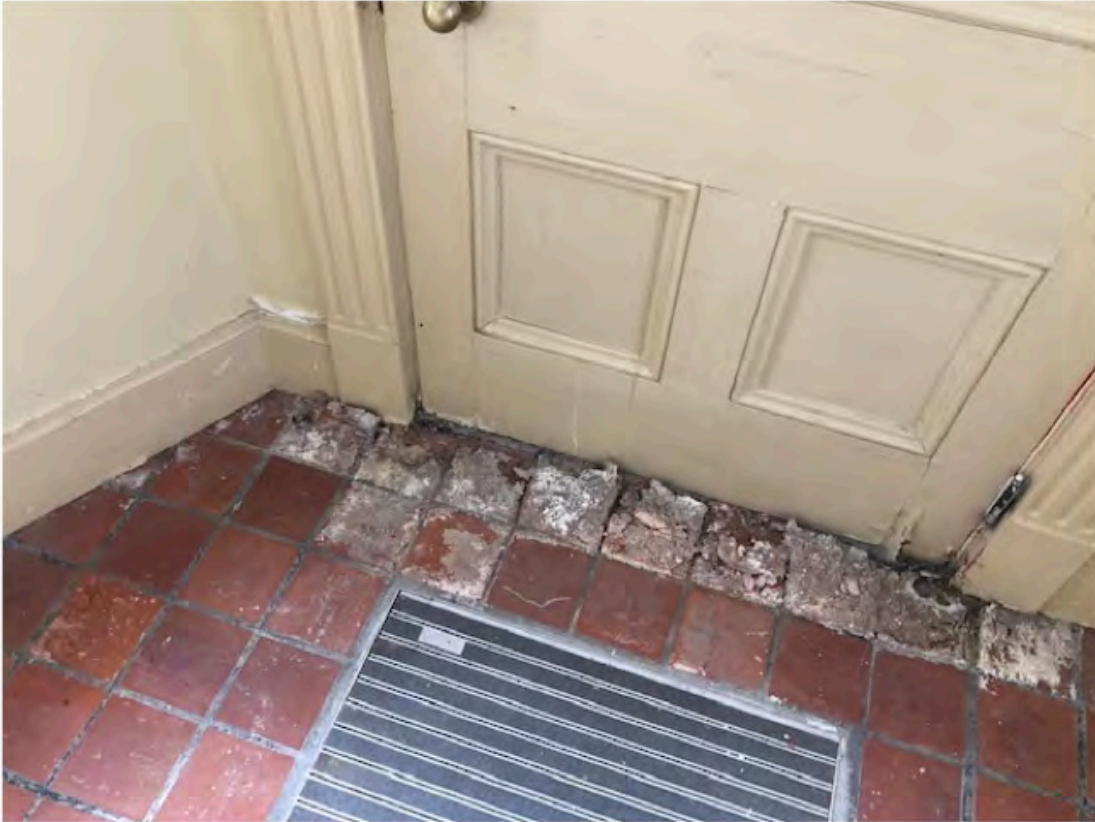
Deteriorated floor tiles - Main entrance vestibule
