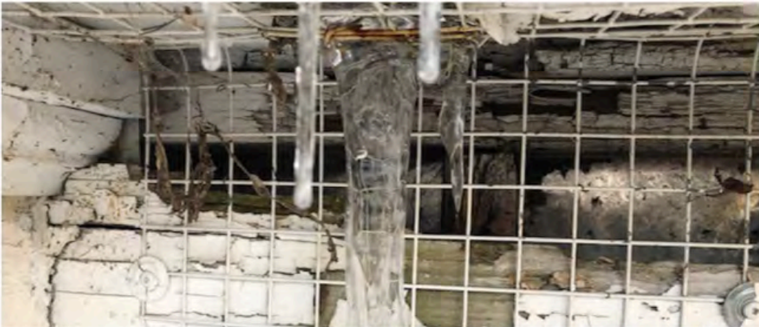
Deteriorated soffit, frieze and siding - West wing north elevation
