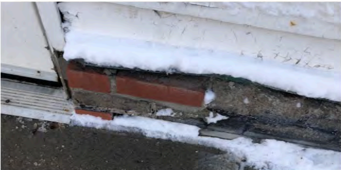
Deteriorated brick at the foundation wall - West wing north elevation
