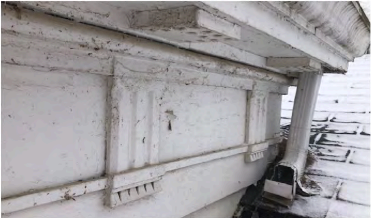
Frieze board with the triglyph detail – Central part of the building north elevation
