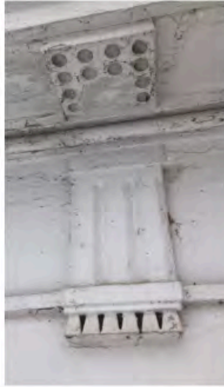
Triglyph detail at the frieze board – Central part of the building south elevation
