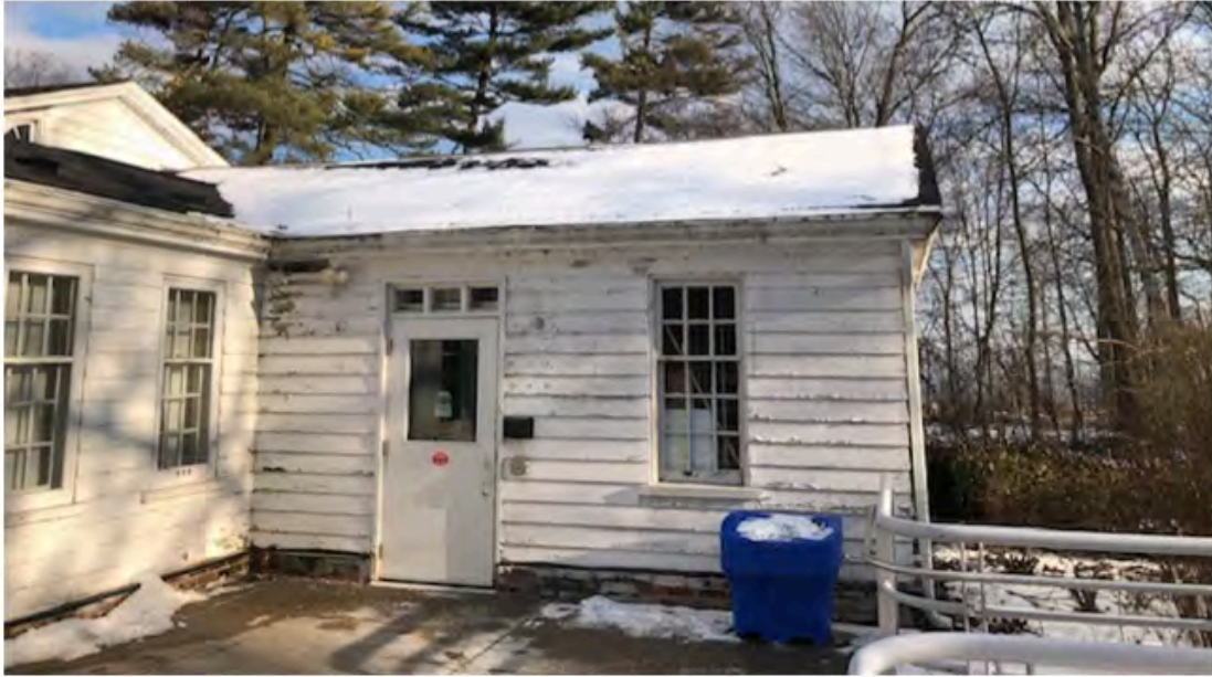
Deteriorated soffit, siding & foundation wall - West wing north elevation
