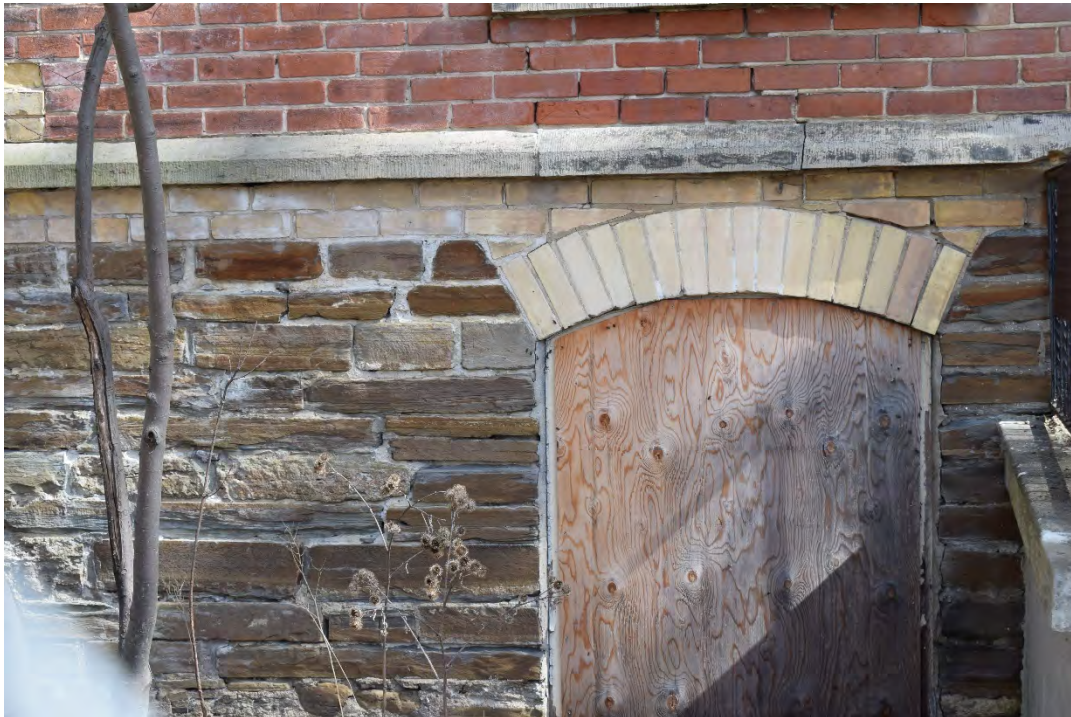
Plate 22: Details of northwest section of basement on front façade, showing rectangular stone block foundation, stone and buff brick band, and buff brick voussoir, looking east.
