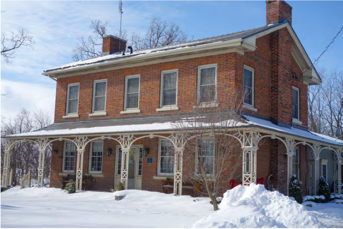
FARMHOUSE – early 19 th century Georgian vernacular farmhouse – brick construction with a centre hall plan, gable roof, end wall chimneys, and a wraparound verandah with wood treillage
