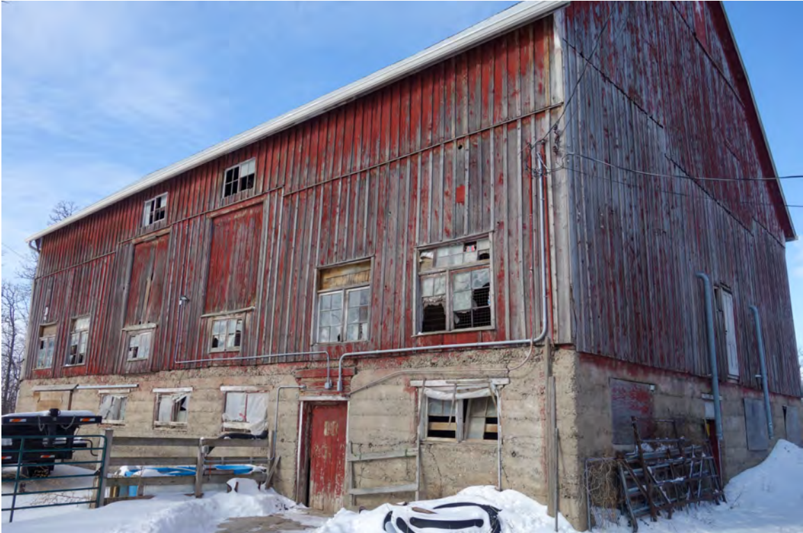
BARN – large timber framed barn with a poured-in-place concrete foundation – concrete may conceal an earlier stone foundation (to be confirmed)
