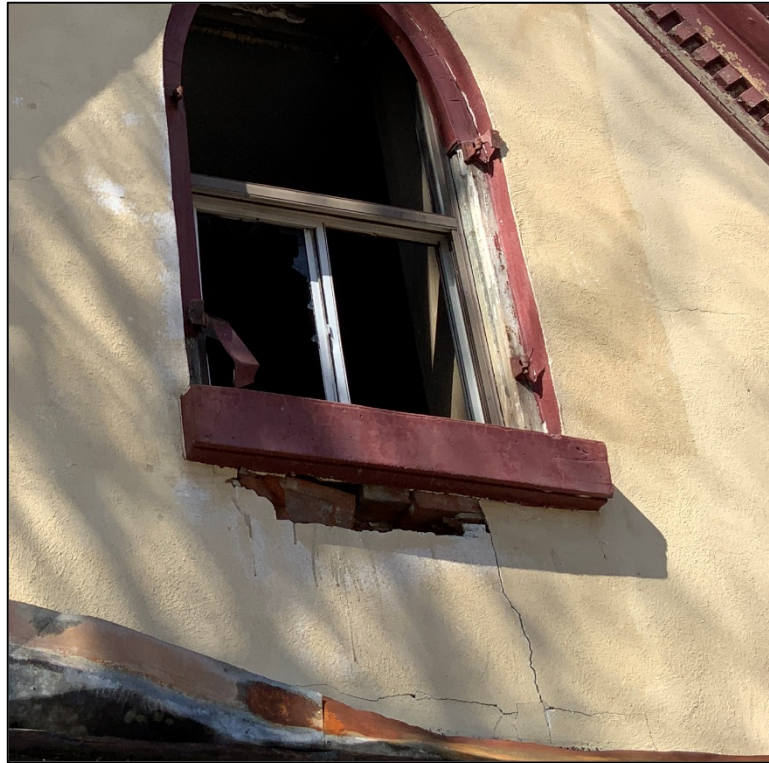
Photograph 2: Destabilization below gable window
