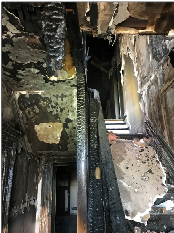
Photograph 7: Fire damage at stair opening
