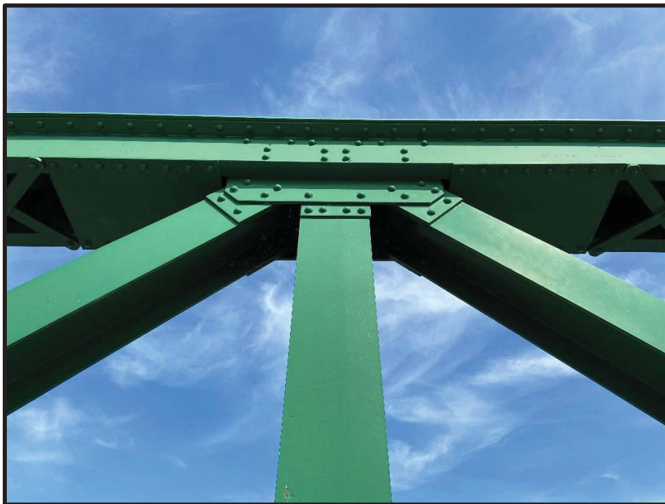
Image 20: Detail of Top Chord Connection, South Side of Old Derry Road Bridge (May 27, 2020; View looking North)
