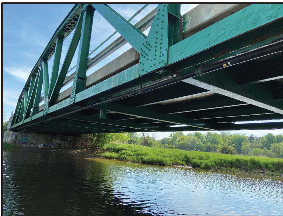
Image 28: Detail of Floor Beams and Stringers, Underside of Old Derry Road Bridge (May 27, 2020; View looking Northeast)
