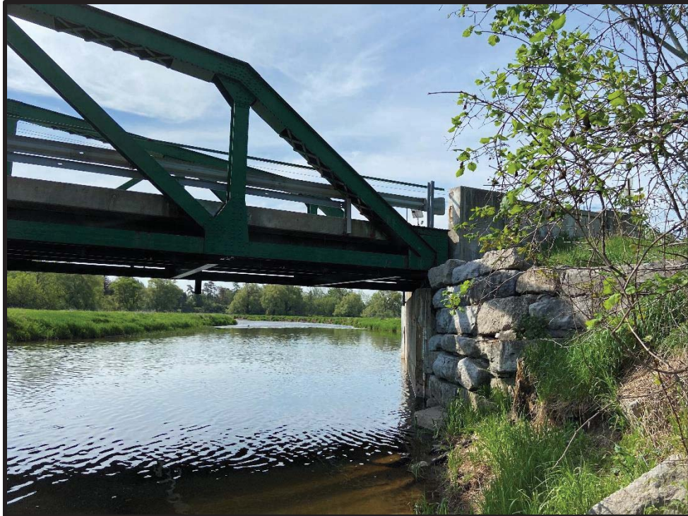
Image 25: Detail of Masonry Gravity Retaining Wall, Northwest Side of Old Derry Road Bridge (May 27, 2020; View looking Southeast)
