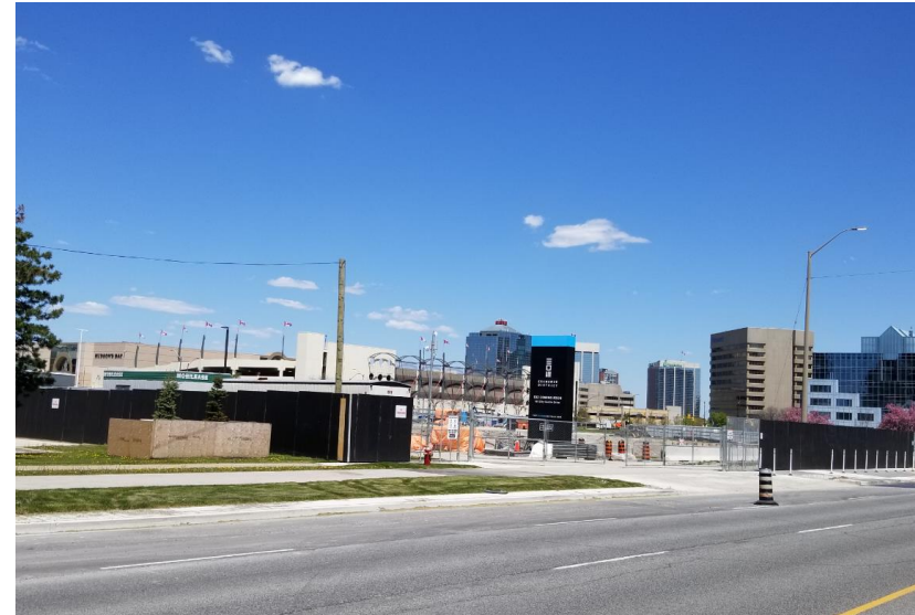
Image of existing conditions facing north from Burnhamthorpe Road West
