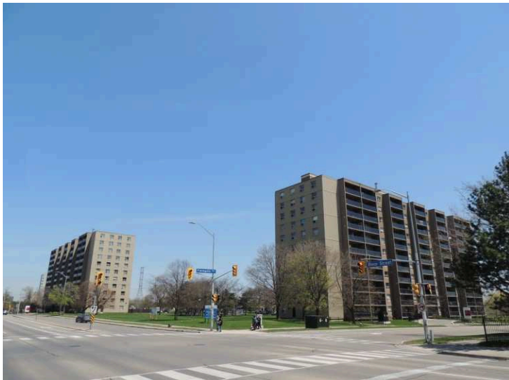
Image of existing conditions
