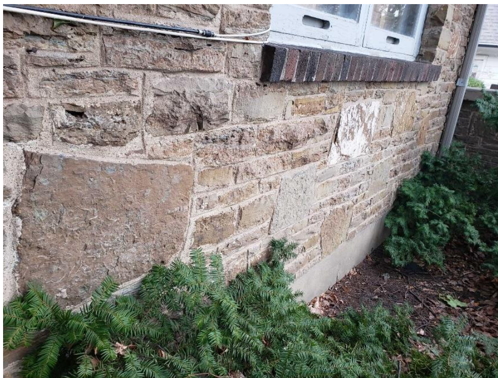
Figure 22 Detail of the front façade of 347 Queen Street South, showing extent of deterioration to the stonework. (Photo by client, Jan. 2021.)
