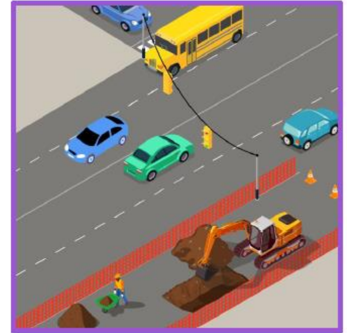
Stage 3: Traffic flips for partial road closure on the other side of Hurontario Street.
