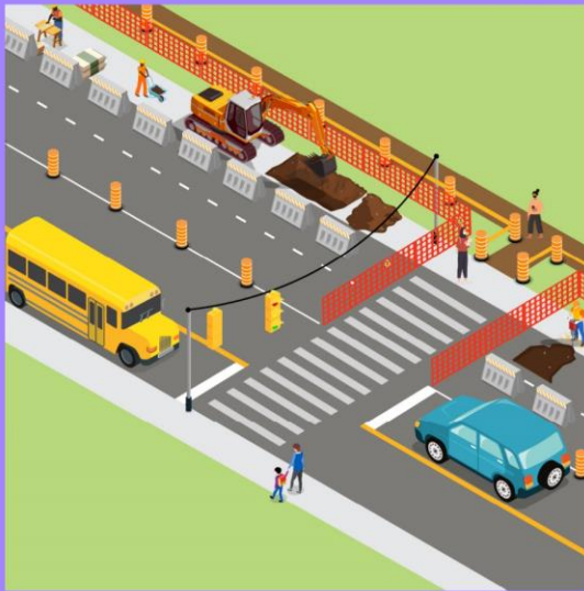
1 REMOVAL OF SIDEWALK
