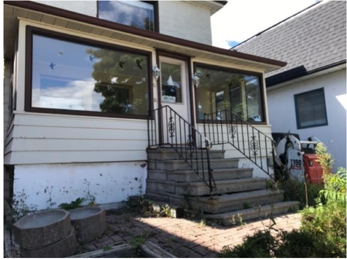
Front of enclosed porch with prefabricated concrete steps and metal railing, plate glass windows photo Picnic Design
