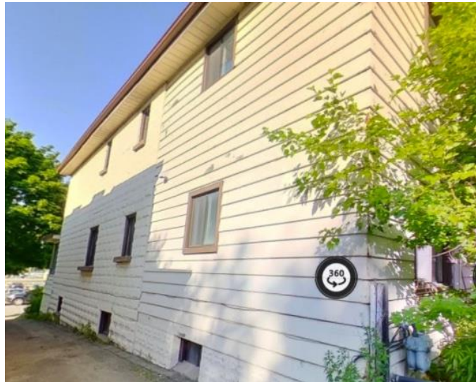
North-west side of house, part concrete block, part aluminum siding, photo Owner
