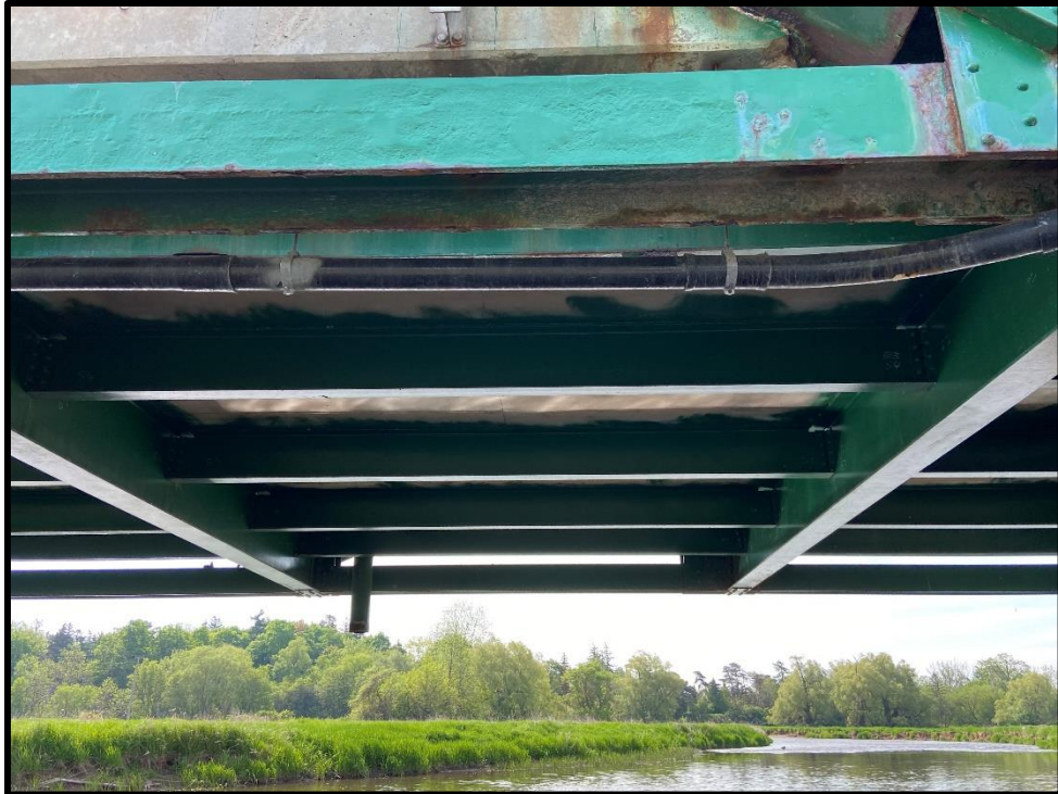
Image 29: Underside Detail of Stringers, Old Derry Road Bridge (May 27, 2020; View looking Southeast)
