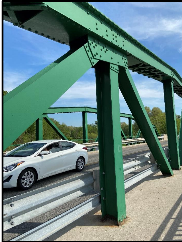
Image 19: Detail of Diagonal and Vertical Members and Rivets, South Side (May 27, 2020; View looking North)
