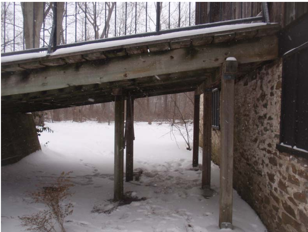
South Portion of the Ramp
