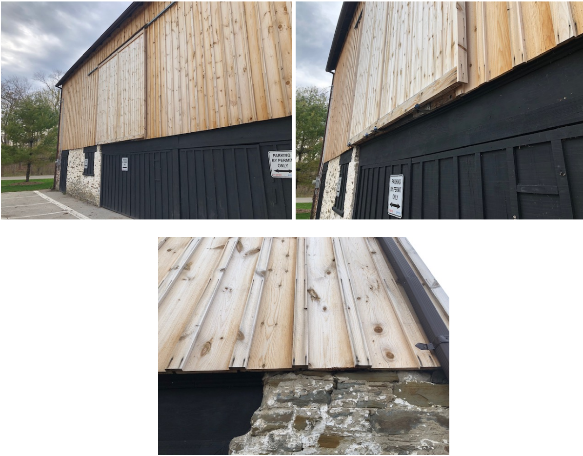
Images of typical board and batten details - recently replaced assembly at the south elevation
