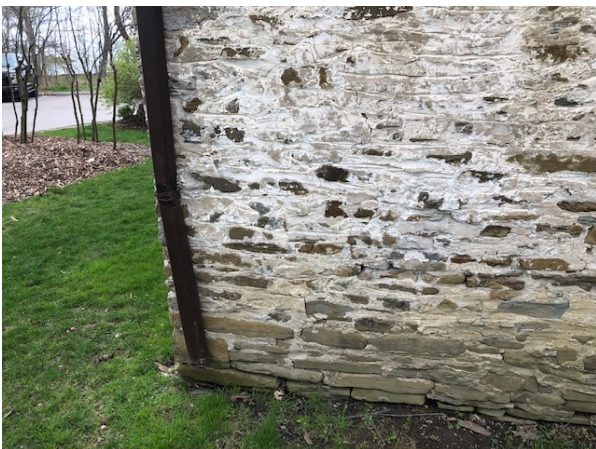
Images of typical mortar joints deterioration found at the east and north elevation
