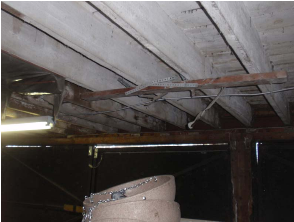
South Bay of Ground Floor Framing (2x10)
