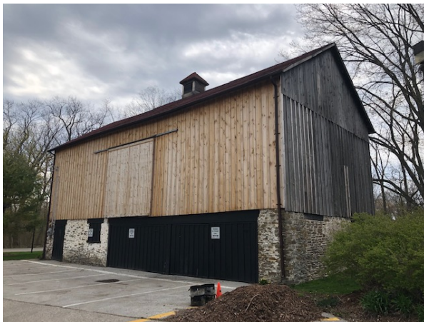
Images of southeast & east elevation – previously replaced boards and battens at south elevation
