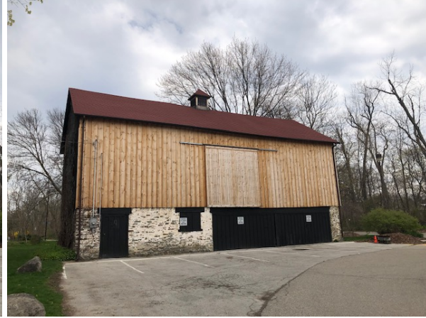
Images of southwest & south elevation – previously replaced boards and battens at south elevation
