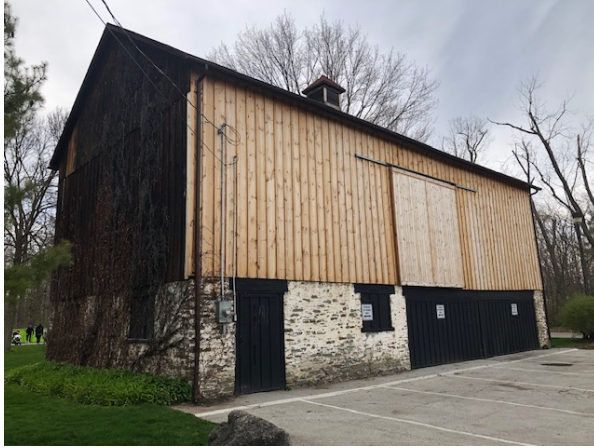
Images of southwest & south elevation – previously replaced boards and battens at south elevation
