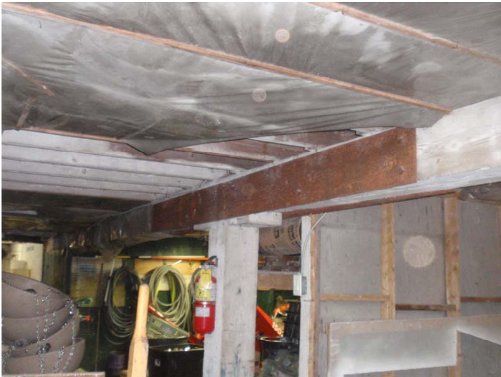
Reinforced Beam of Ground Floor Framing
