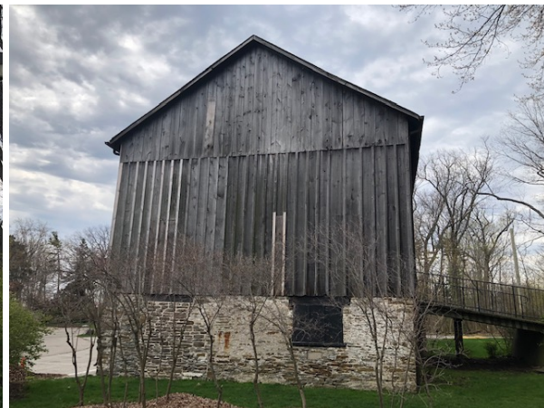
Images of southeast & east elevation – previously replaced boards and battens at south elevation
