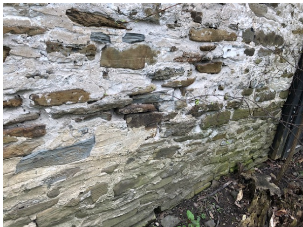
Images of typical mortar joints deterioration found at the east and north elevation
