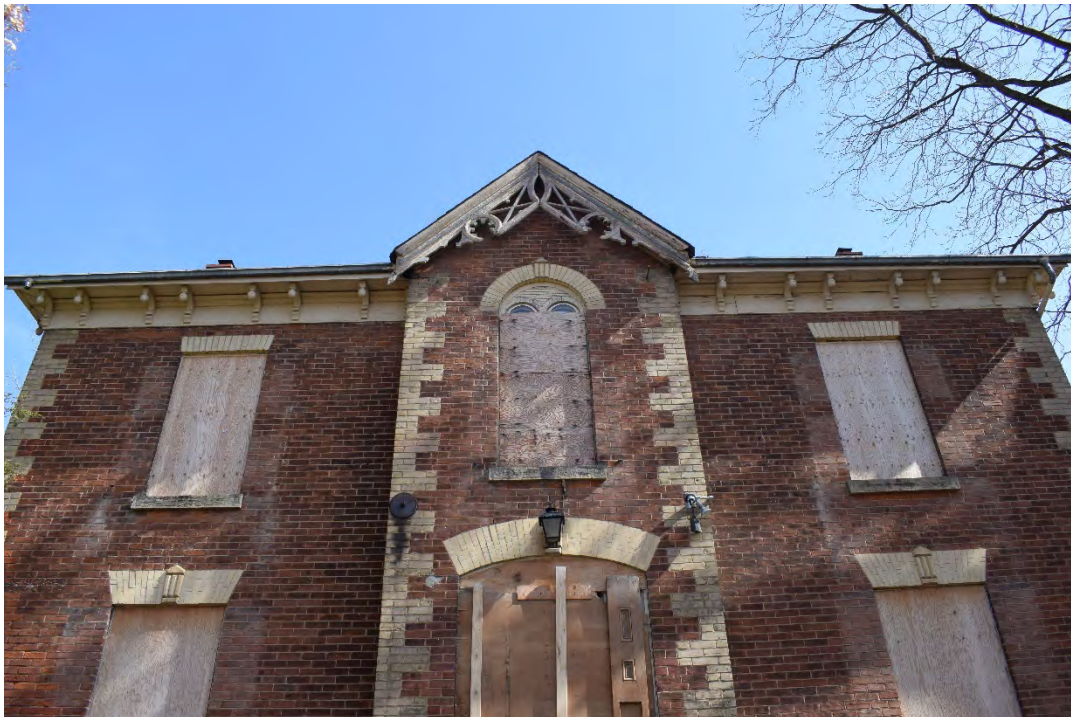
Plate 20: Details of second storey showing cornice, brackets, bargeboard, and second storey windows, looking east.
