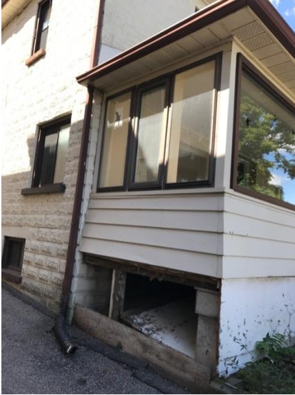
Side of enclosed porch, aluminum siding, concrete foundation wall, photo Picnic Design
