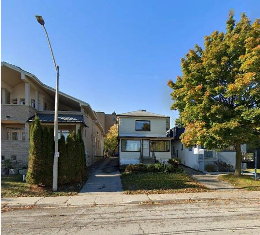
Existing conditions, showing the relationship to adjacent properties. The original windows have been replaced with large windows, the roof line is original. photo Google Earth
