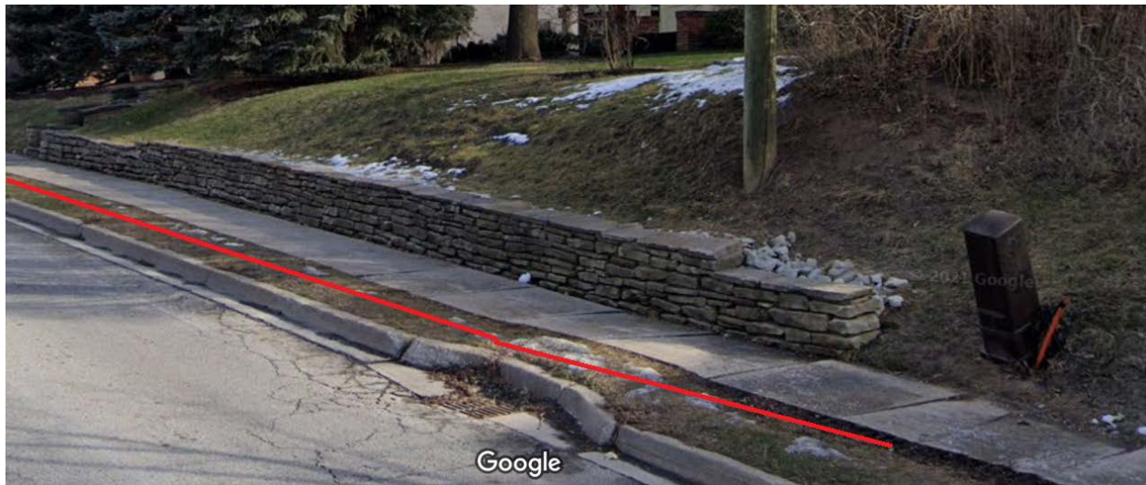
Area of widened sidewalk, facing east. Proposed sidewalk width illustrated in red
