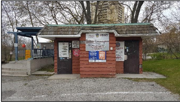
Figure 55: Marina Park Washroom north elevation (ASI 2020)
