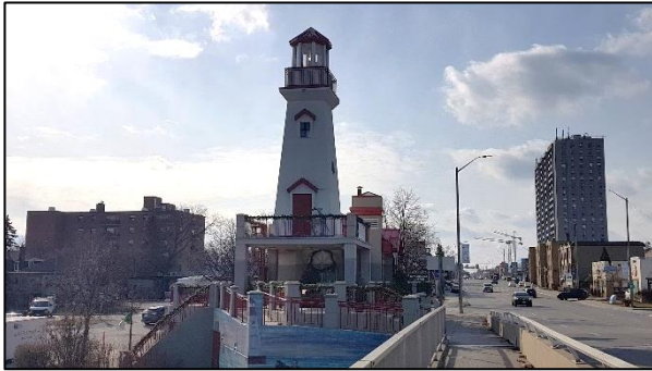
Figure 37: Port Credit Lighthouse and Front Street Pumping Station, east elevation (ASI)
