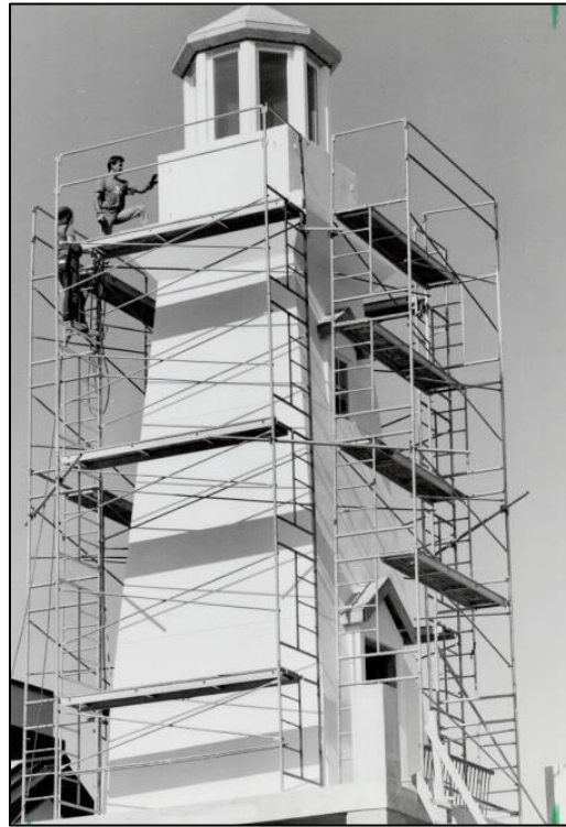
Figure 15: Construction of the Port Credit Lighthouse in 1991 (Toronto Public Library tspa_0106743f)
