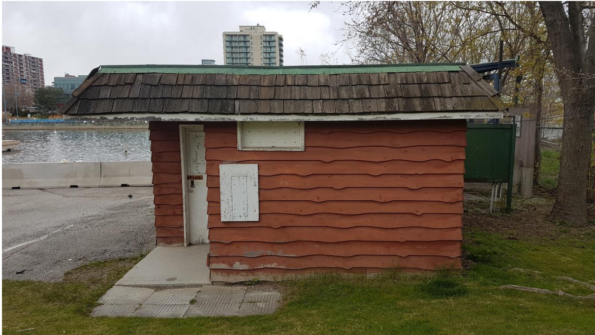
Marina Park Washroom, west elevation (ASI 2020)
