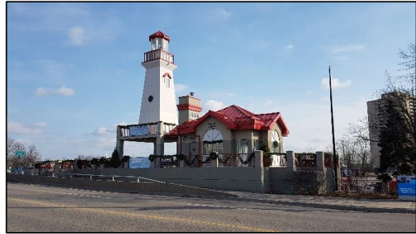
Figure 38: Port Credit Lighthouse and Front Street Pumping Station, north elevation (ASI 2019)
