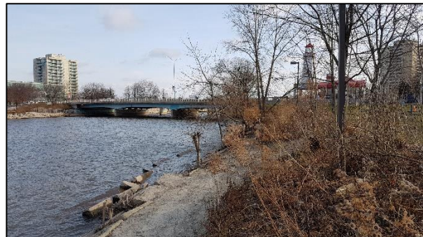
Figure 27: Port Credit Memorial Park West shoreline condition (ASI 2019)
