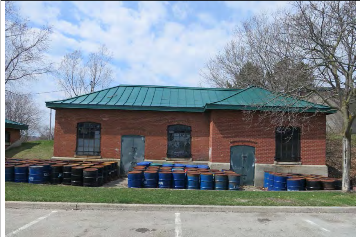
6.3 South elevation, pumping station
