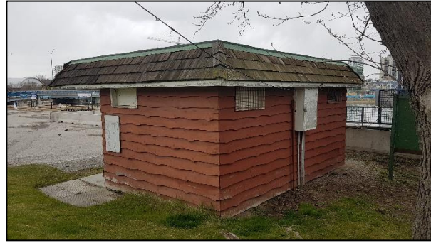
Figure 60: Marina Park Washroom west and south elevation (ASI 2020)
