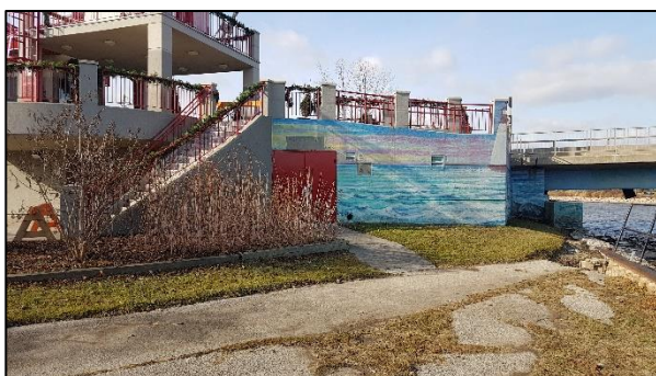
Figure 43: Pumping Station Access and staircase to the patio space (ASI 2019)
