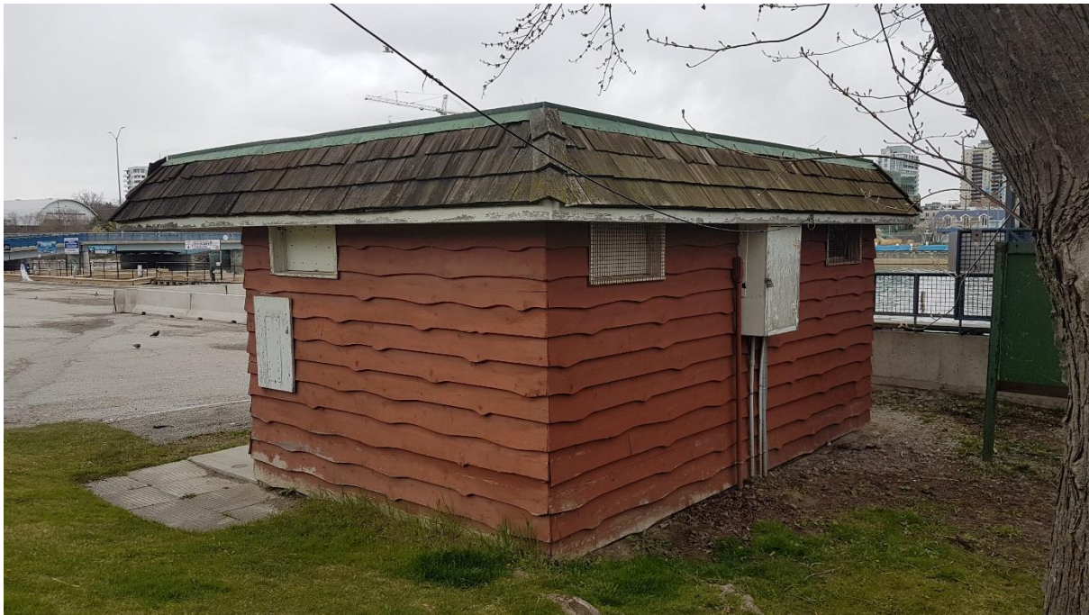
Marina Park Washroom, west and south elevations (ASI 2020)
