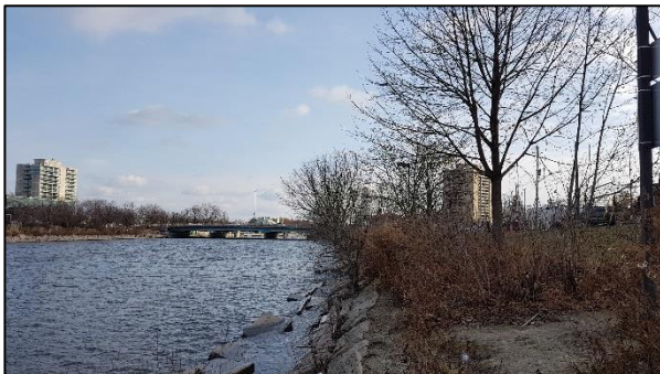
Figure 26: Port Credit Memorial Park West shoreline condition (ASI 2019)
