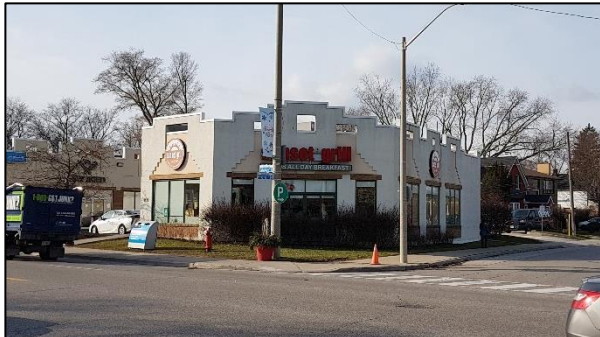
Figure 84: 102 Lakeshore Road West (ASI 2019)
