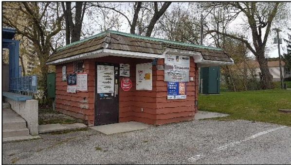
Figure 57: Marina Park Washroom north and east elevation (ASI 2020)
