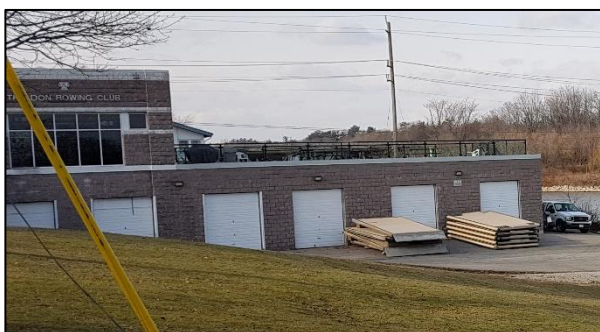
Figure 22: Don Rowing Club, south elevation (ASI 2019)
