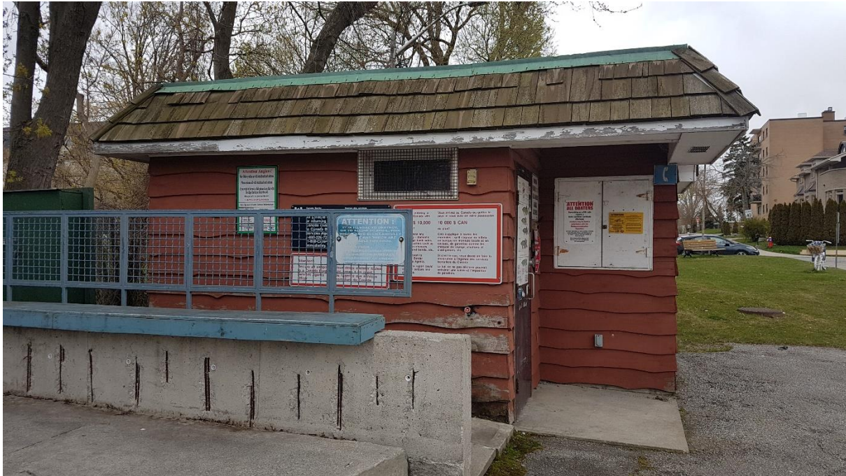
Marina Park Washroom, east elevation (ASI 2020)
