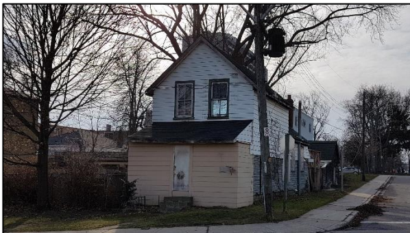
Figure 83: 16 Front Street North (ASI 2019)
