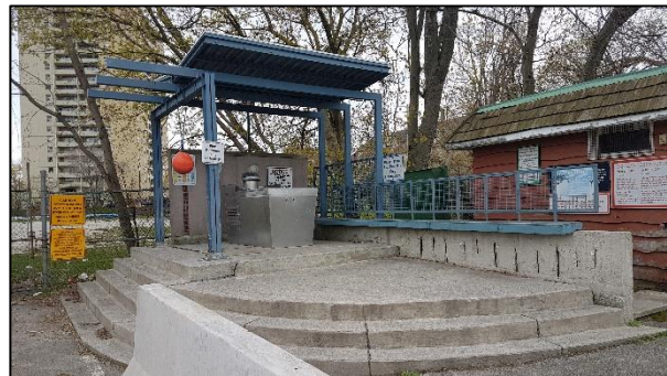
Figure 62: Fish cleaning station (ASI 2020)
