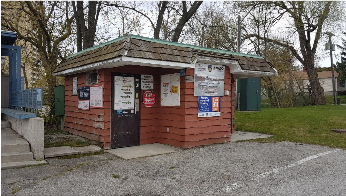
Marina Park Washroom, north and east elevations
