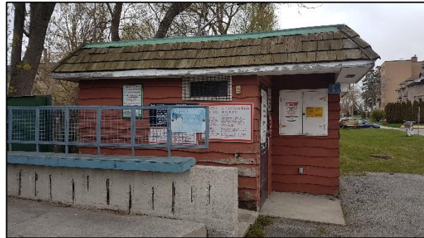
Figure 58: Marina Park Washroom east elevation (ASI 2020)
