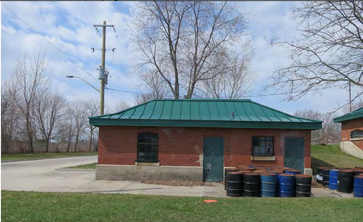
6.2 South elevation, pumping station, 2017/05/08
