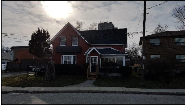
Figure 81: 10 Front Street North (ASI 2019)
