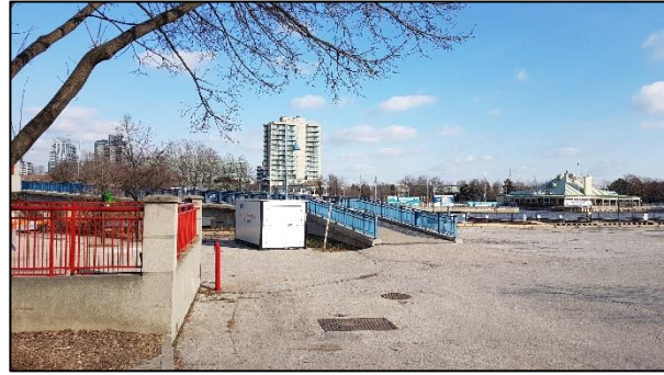
Figure 46: Marina Park pedestrian ramp (ASI 2019)
