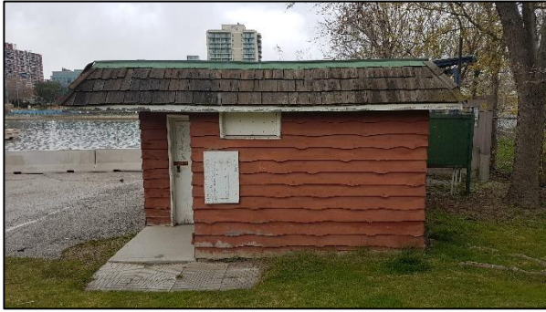
Figure 59: Marina Park Washroom west elevation (ASI 2020)
