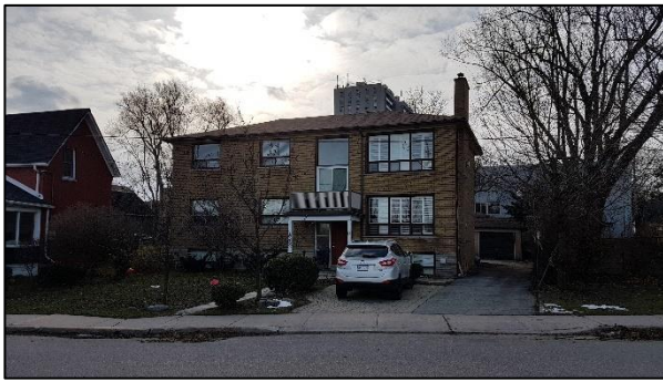
Figure 82: 14 Front Street North (ASI 2019)
