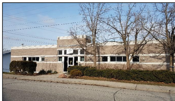
Figure 21: Don Rowing Club, west elevation (ASI 2019)
