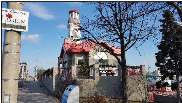
Figure 39: Port Credit Lighthouse and Front Street Pumping Station, west elevation (ASI 2019)
