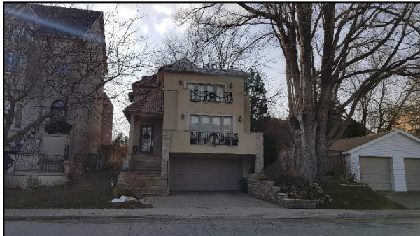
Figure 76: 24 Front Street South (ASI 2019)
