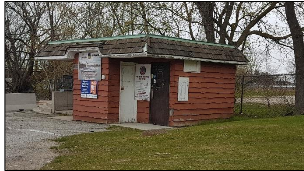
Figure 56: Marina Park Washroom north and west elevation (ASI 2020)
