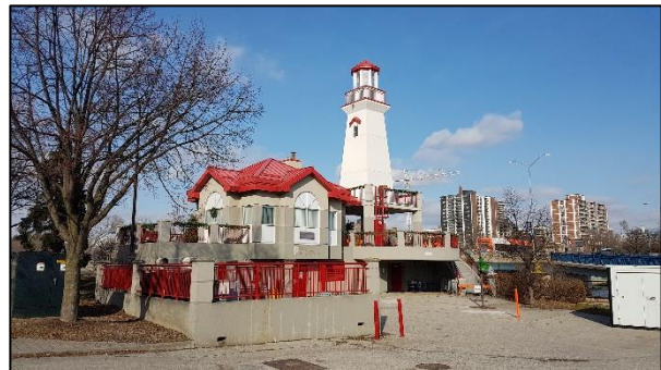
Figure 40: Port Credit Lighthouse and Front Street Pumping Station, south elevation (ASI 2019)
