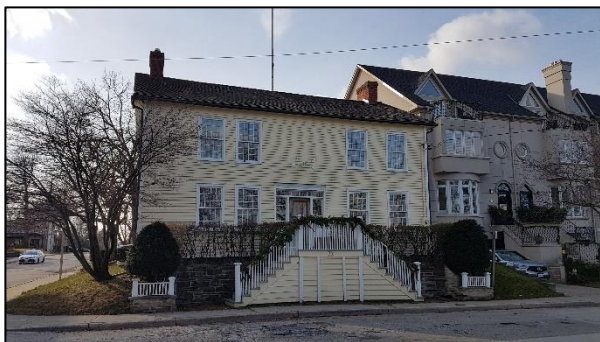
Figure 78: 32 Front Street South (ASI 2019)
