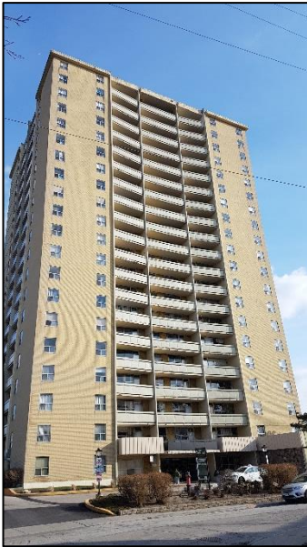
Figure 79: 35 Front Street South (ASI 2019)
