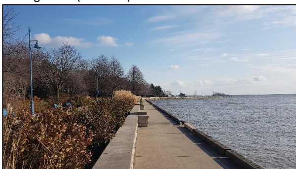
Figure 93: 18 Stavebank Road South (J.J. Plaus Park), looking south (ASI 2019)
