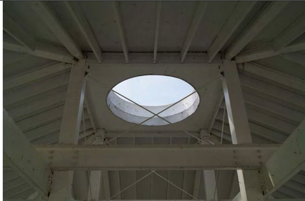
6.2 Detail, shade structure, 2018/05/14
