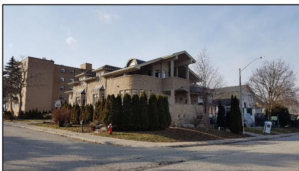
Figure 75: 16 Front Street South (ASI 2019)
