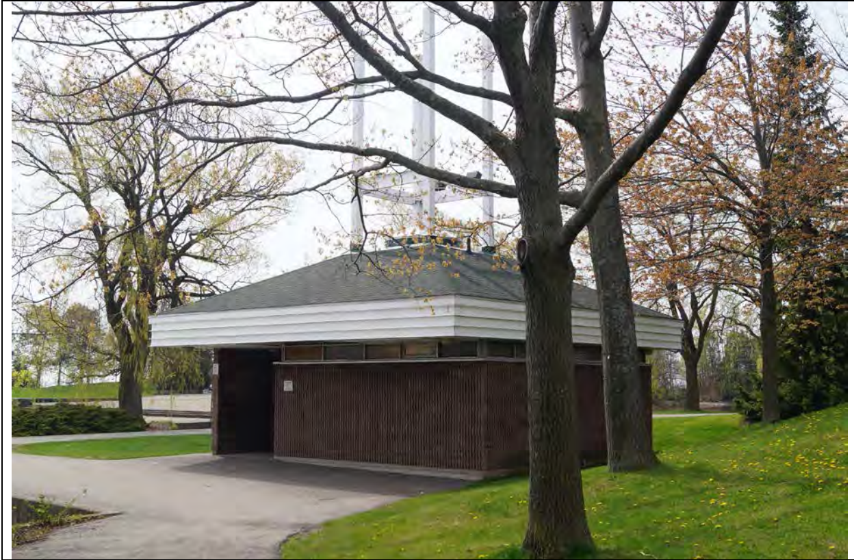
6.3 Northeast corner, public washrooms, 2018/05/14
