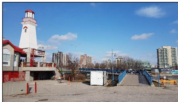
Figure 42: Port Credit Lighthouse and Front Street Pumping Station, servicing area and adjacent Waterfront Trail bridge ramp (ASI 2019)
