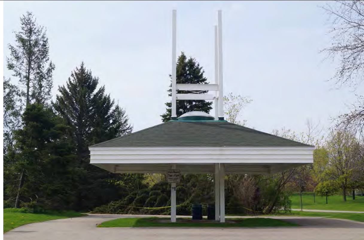
6.1 North elevation, shade structure, 2018/05/14
