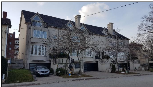
Figure 77: 28 Front Street South (ASI 2019)
