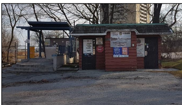
Figure 51: Marina Park washroom and fish cleaning station (ASI 2019)
