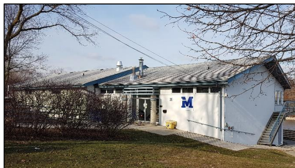
Figure 18: Mississauga Canoe Club, west and south elevations (ASI 2019)
