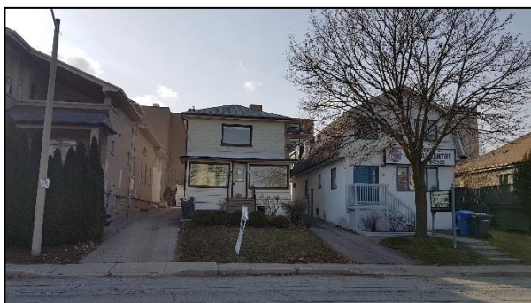
Figure 74: 14 Front Street South (ASI 2019)
