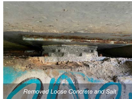
Power Washing of Bearing Seats on Burnhamthorpe Road West Structures
