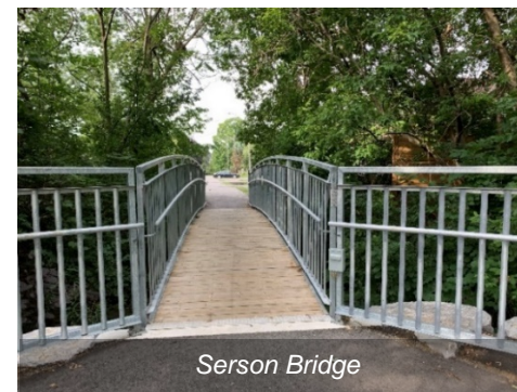
Replacement in 2019 with Galvanized Steel Structure and Kebony Wood Decking
