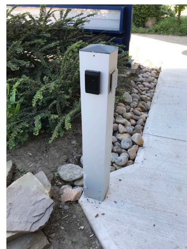
New Card Access & Door Operator Pedestal along barrier free access path
