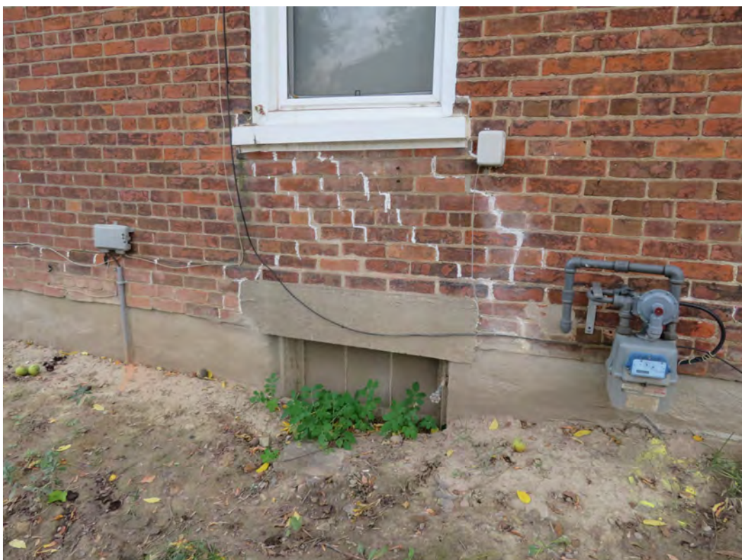
SIDE ELEVATION – masonry condition issues
