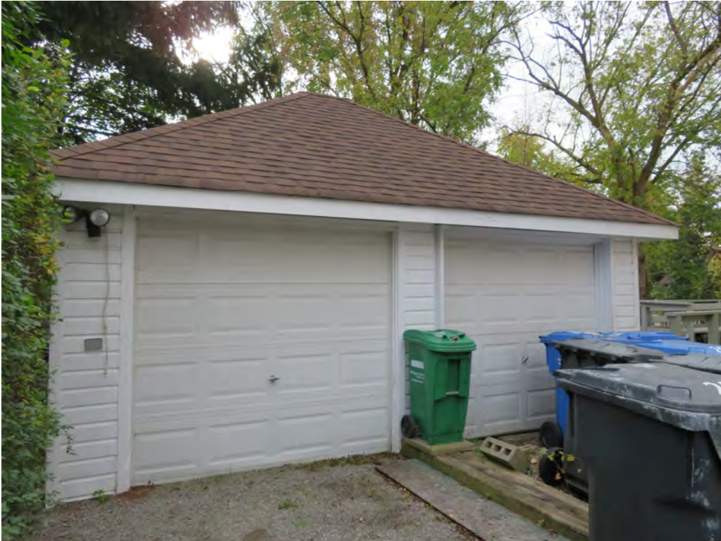
GARAGE – FRONT ELEVATION - frame garage with vinyl cladding
