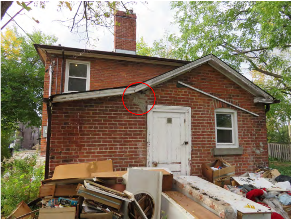
1-STOREY REAR ADDITION – to be demolished – masonry condition issues above the door
