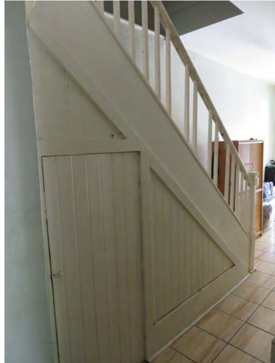
MAIN STAIRCASE – narrow staircase with a crude newel post – plain skirting board & tongue & groove paneling
