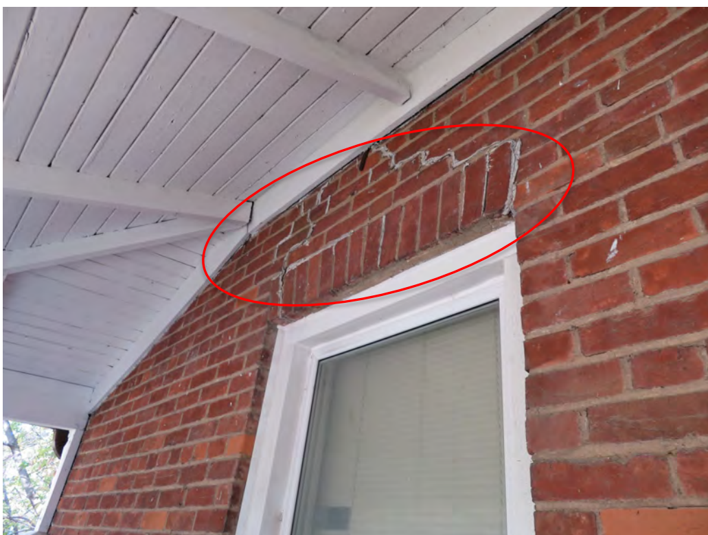
FRONT ELEVATION – masonry issues above window
