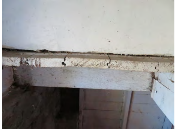
STAIRS TO BASEMENT – tongue and groove floorboards are thick, approx. 1"
