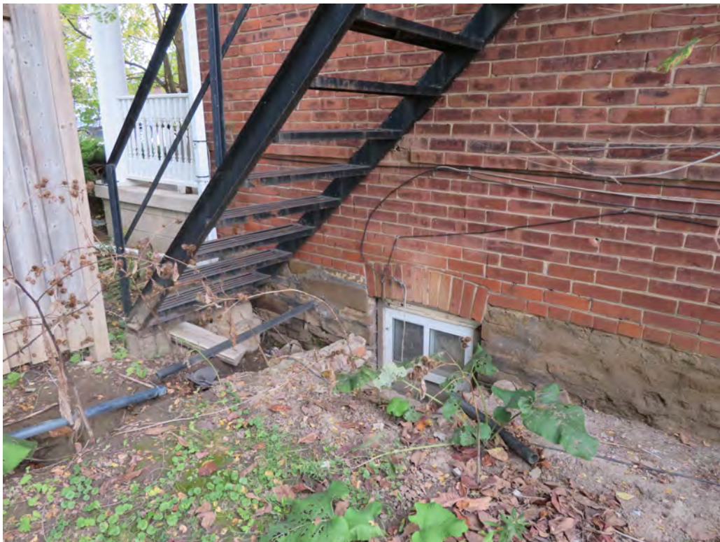
SIDE ELEVATION – basement window with brick soldier arch – rubble stone foundation
