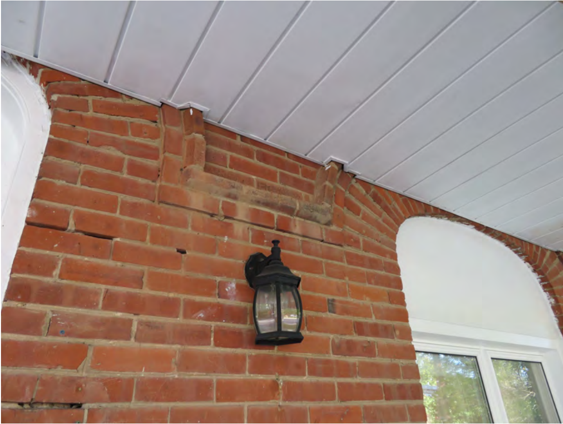
FRONT ELEVATION – the porch has been carefully installed so that the raised brick banding is intact
