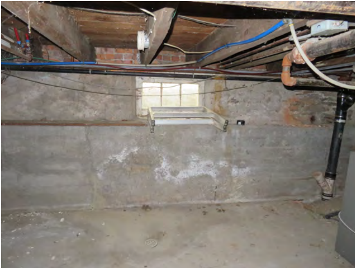
BASEMENT – rubble stone foundation appears to have been underpinned – floor joists are widely spaced, approx. 24"
