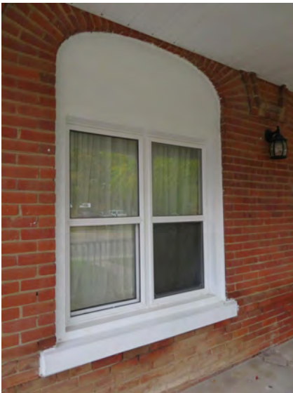
MAIN ELEVATION – modern vinyl window – the window frame and sill have been clad with aluminum
