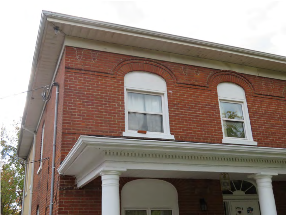
MAIN ELEVATION – arched window openings with a brick soldier arch and raised brick banding – modern vinyl windows have been installed in the arched masonry openings and the arch has been filled in with plywood
