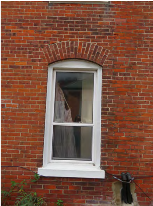
SIDE ELEVATION – segmentally arched window opening with a brick soldier arch – a modern vinyl window with a flat head has been installed
