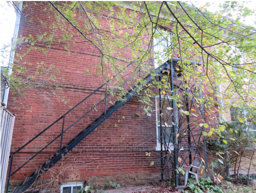
SIDE ELEVATION – this elevation faces Victoria Street and has the same raised brick banding as the main elevation – the elevation that faces the driveway is plainer, without any decorative brickwork – the top of the Credit Valley stone foundation is visible on this elevation – the metal fire escape was installed before 1990
