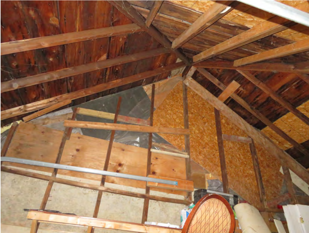
GARAGE – INTERIOR – later partition wall down the middle and original roof framing dating from the early to mid-20 th century
