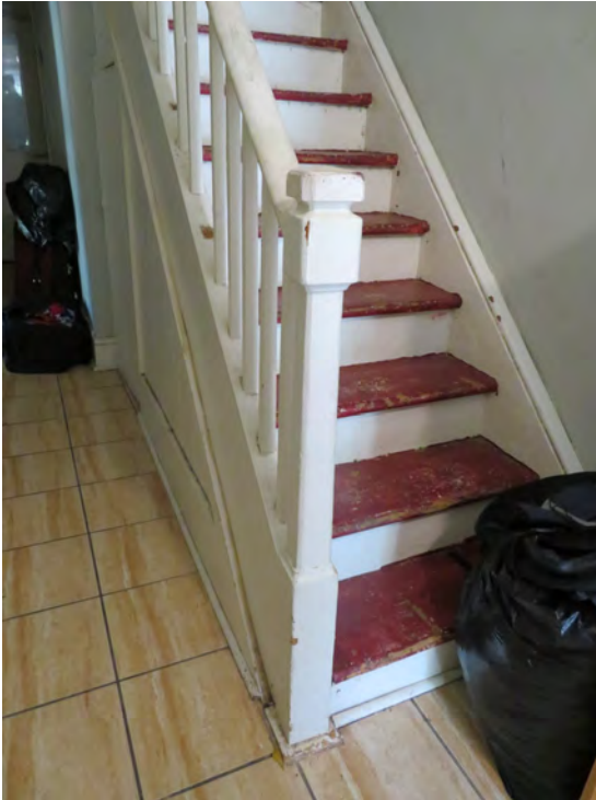
MAIN STAIRCASE – narrow staircase with a crude newel post – plain skirting board & tongue & groove paneling
