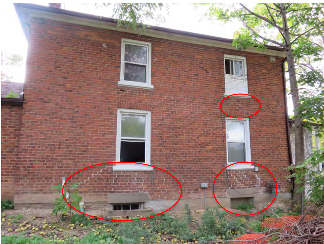
SIDE ELEVATION – foundation settlement and sheer cracks
