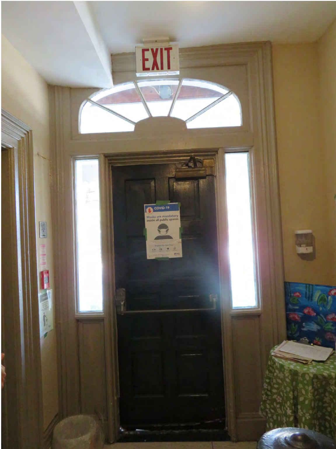
INTERIOR Historic portion - original sidelights and fanlight transom – modern security door has been installed – modern ductwork partially covers the fanlight
