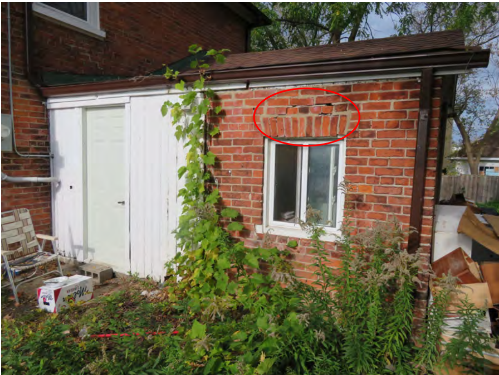
1-STOREY REAR ADDITION – to be demolished – door has been modified – window has been replaced – masonry condition issues above the window
