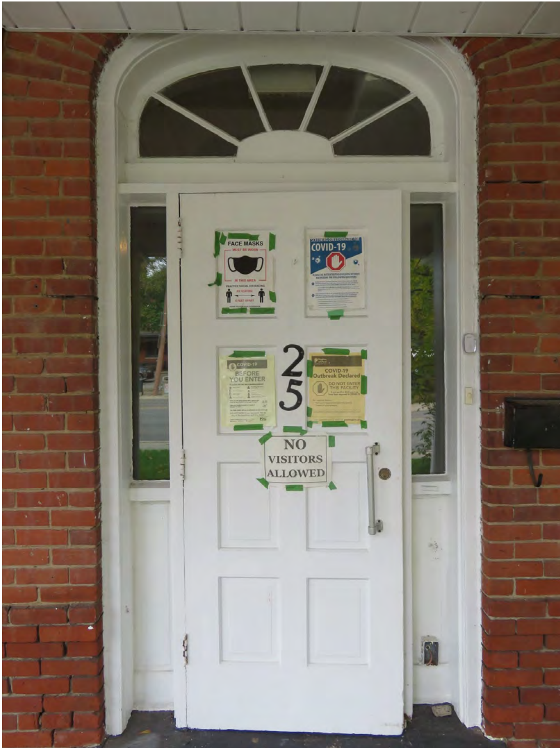
FRONT DOOR – a modern door has been installed but the original fanlight and sidelights are intact – the roof of the porch overlaps the top of the arch
