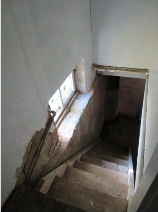
STAIRS TO BASEMENT – tongue and groove floorboards are thick, approx. 1"
