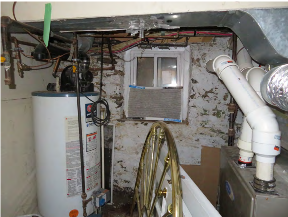
INTERIOR Historic portion basement – furnace room – rubblestone foundation
