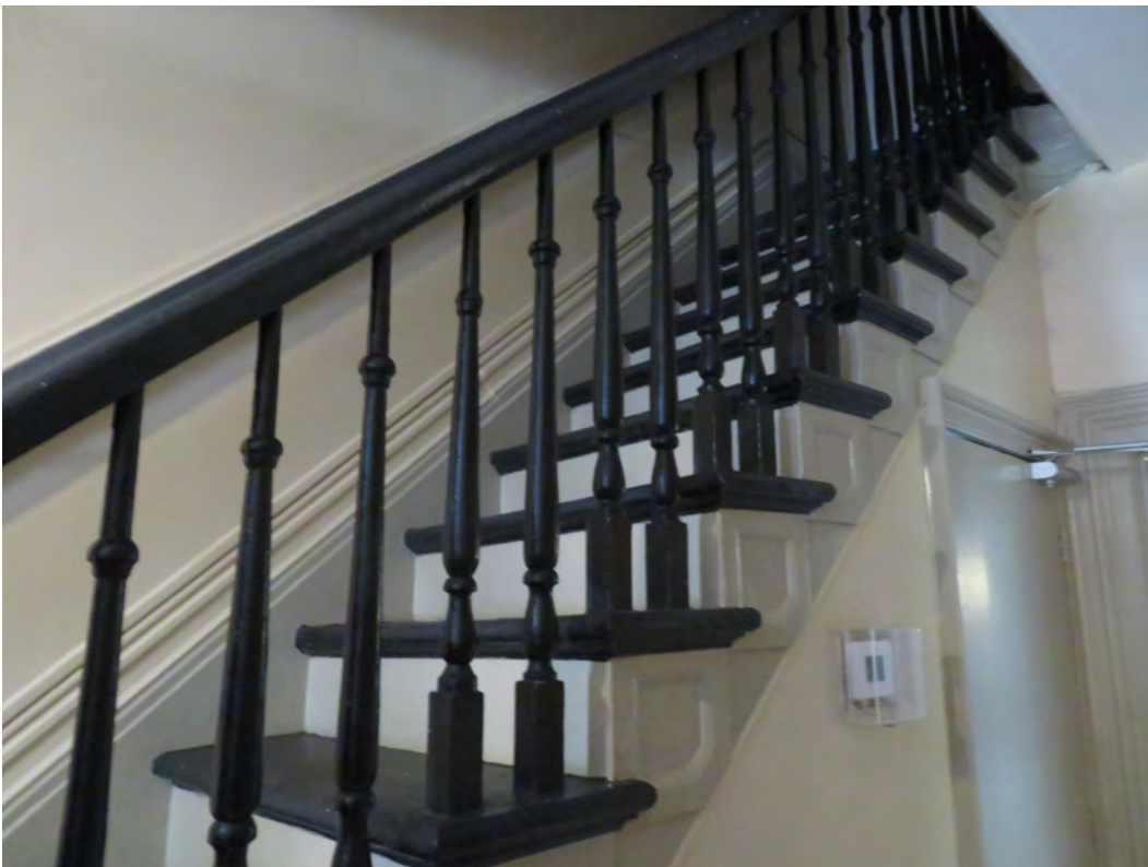
INTERIOR Historic portion – original stairs to 2 nd floor with curved handrail and turned balusters
