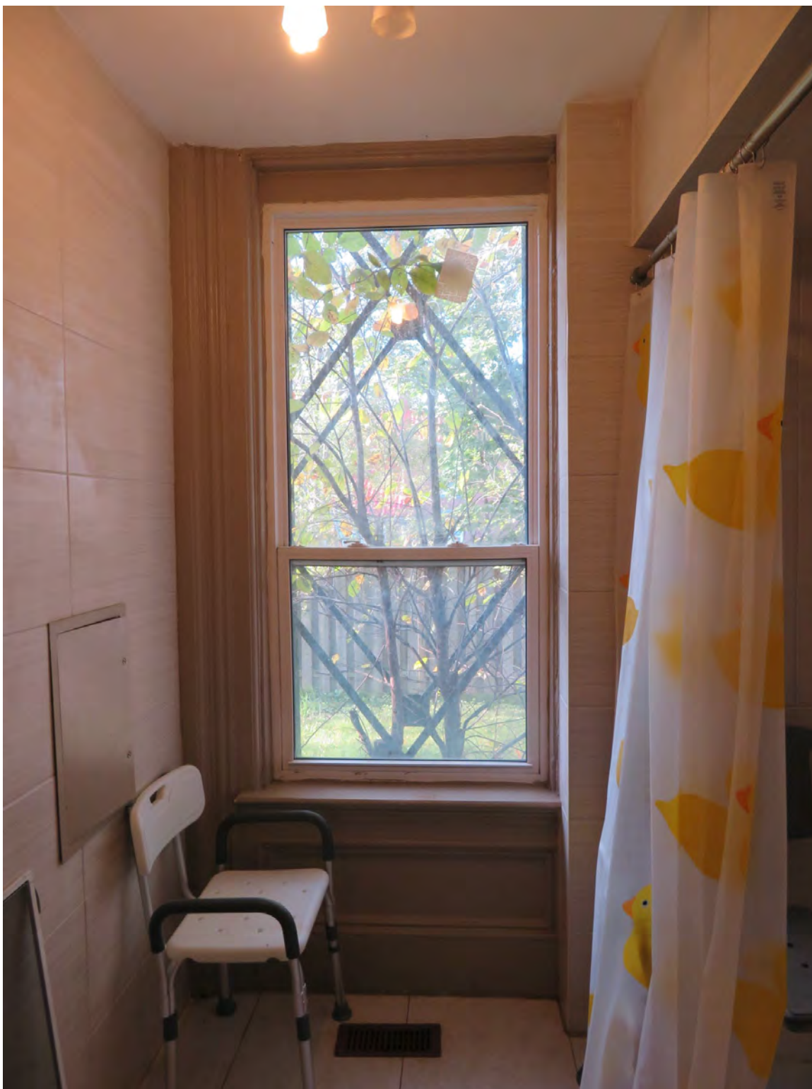
INTERIOR Historic portion – 1 st floor bathroom – original window trim with paneled dado
