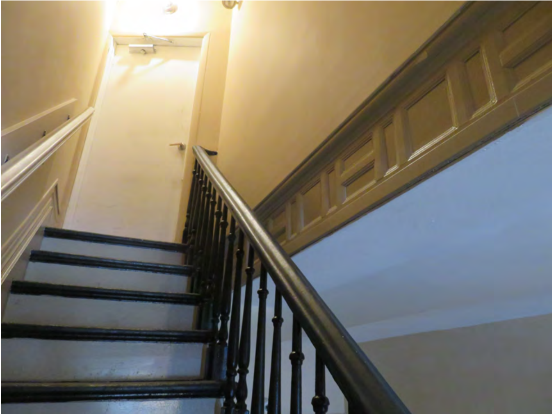
INTERIOR Historic portion – original stairs to 2 nd floor (landing has been enclosed and upper railing removed)
