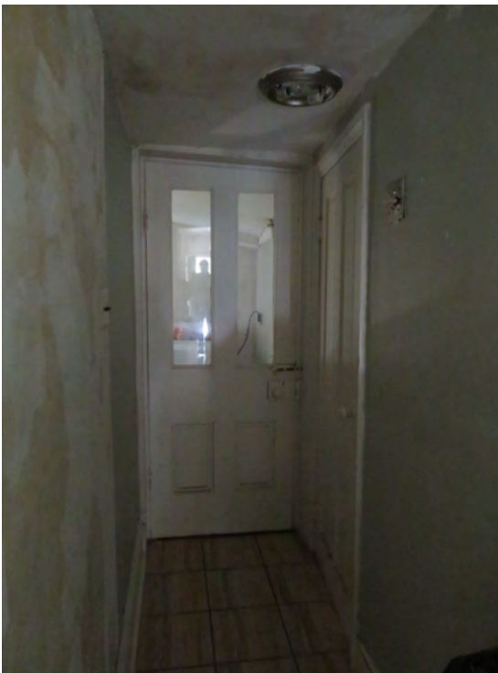
1 st floor HALLWAY & PARLOUR – wood doors with 4 panels are in poor condition - modern drop ceilings installed
