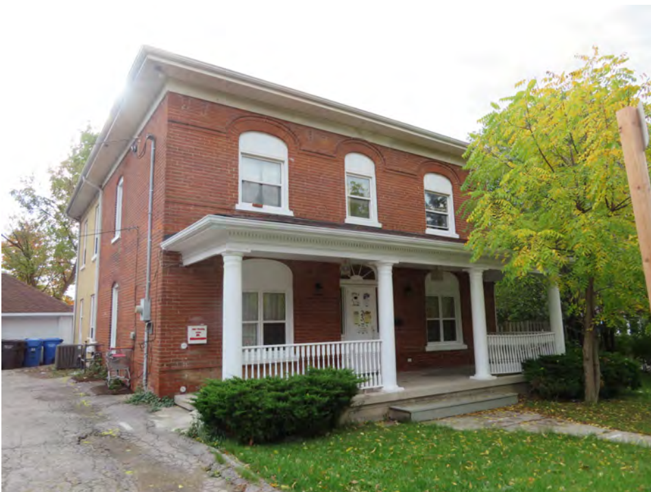
FRONT & SIDE ELEVATION – porch added after 1990 – original arched windows replaced with modern units and the arches infilled with plywood
